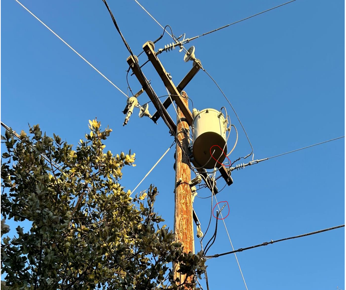
Figure 4 – Troubleshooter #1 removed the two connectors from the transformer jumpers and made the area safe. Picture taken by the troubleshooter on September 3, 2024.
