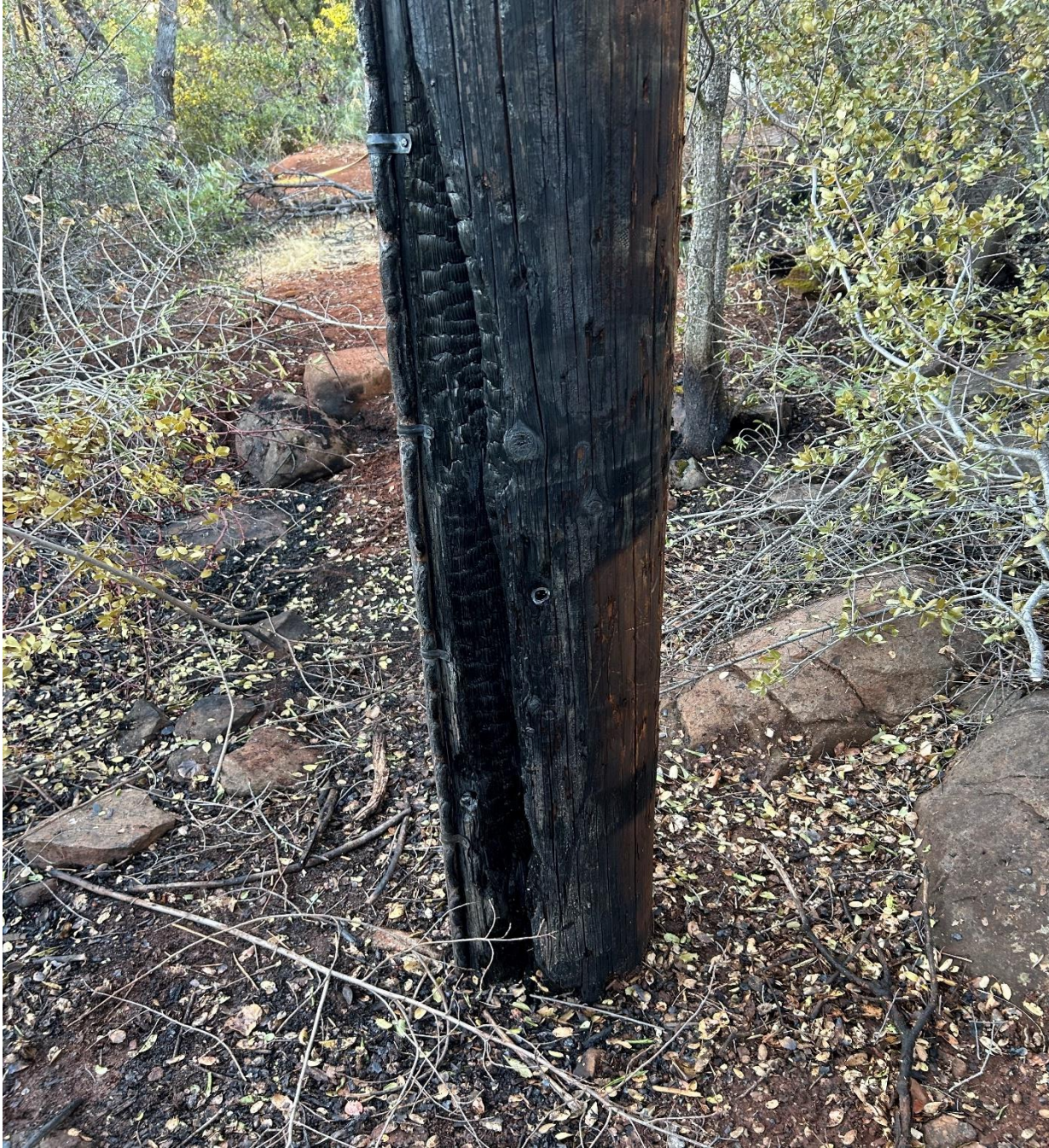
Figure 5 The secondary service hot-leg connector failed from overloading on the service which caused arcing and burned vegetation below at the base of SAP Pole ID # 101485155. Picture taken by the troubleshooter on September 3, 2024.
