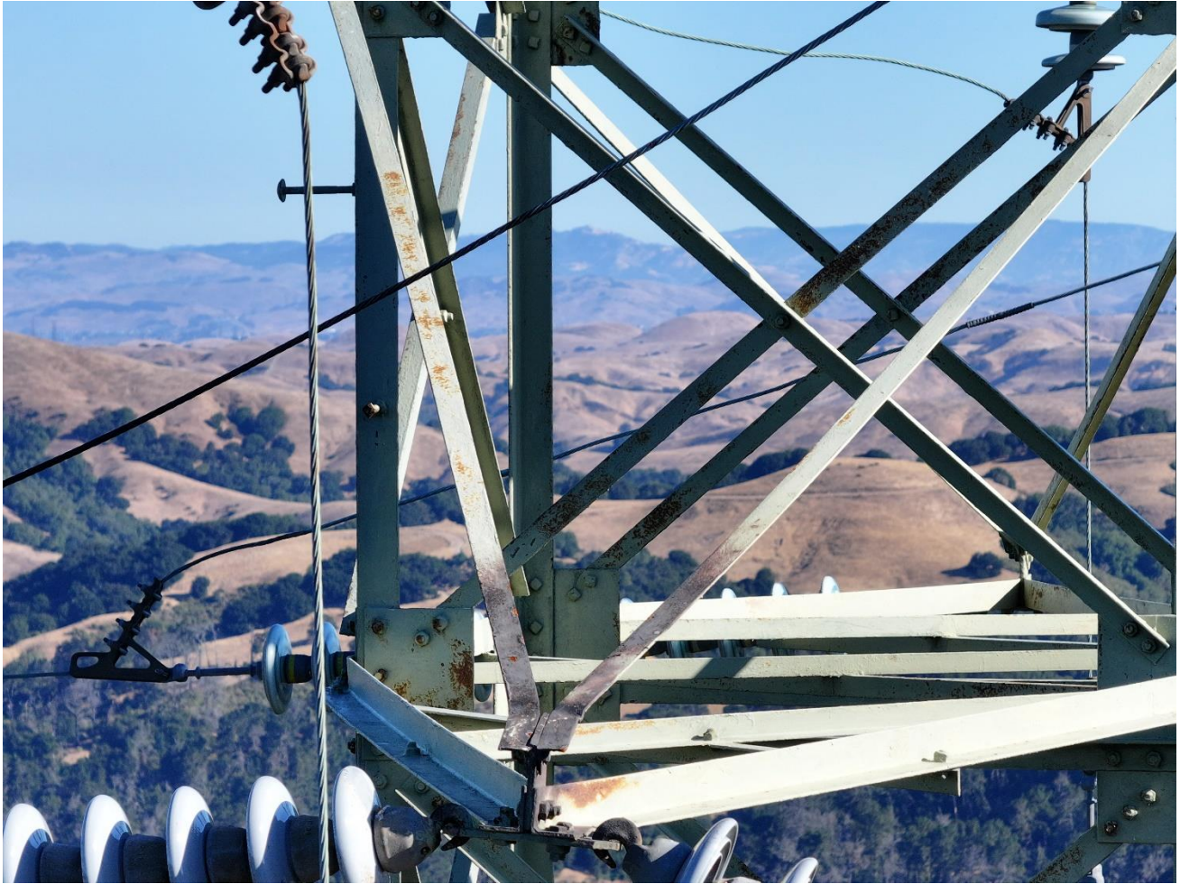
Figure 6 Arc marks on the corner of the steel crossarm (bottom center of photo). Drone photo taken by Ignition Investigator on September 12, 2024.
