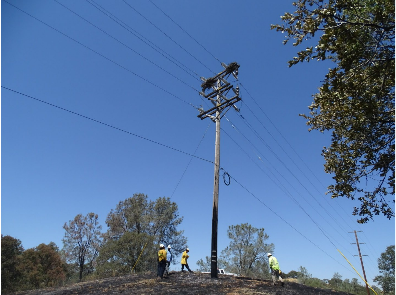
Figure 3 Pole #1 - Incident Location - Bird nest on both sides of upper crossarm. Photo taken by troubleshooter on August 7, 2024.
