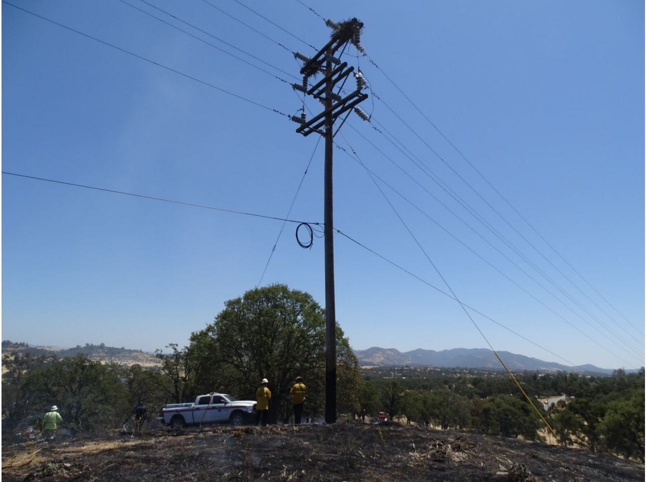
Figure 2 Pole #1 - Incident Location - Bird nest on both sides of upper crossarm. Photo taken by troubleshooter on August 7, 2024.
