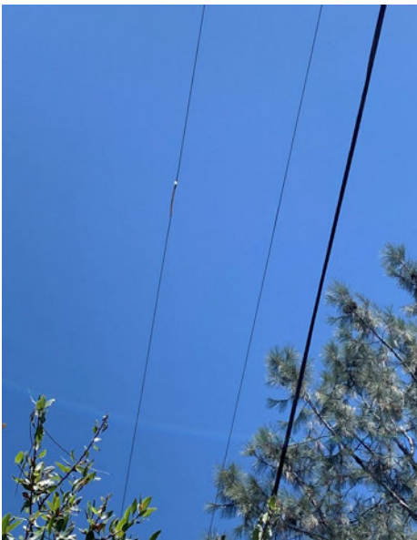
Photo 7: taken by vegetation management crew, post incident, showing repair splice
