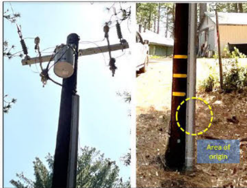
Figure 7 - The pole ignition likely resulted from the failure of a secondary riser involving 1/0 aluminum conductors. A visual inspection of the conductor revealed melting patterns on two hot legs, leading to the breakage of aluminum strands near the ground line.
