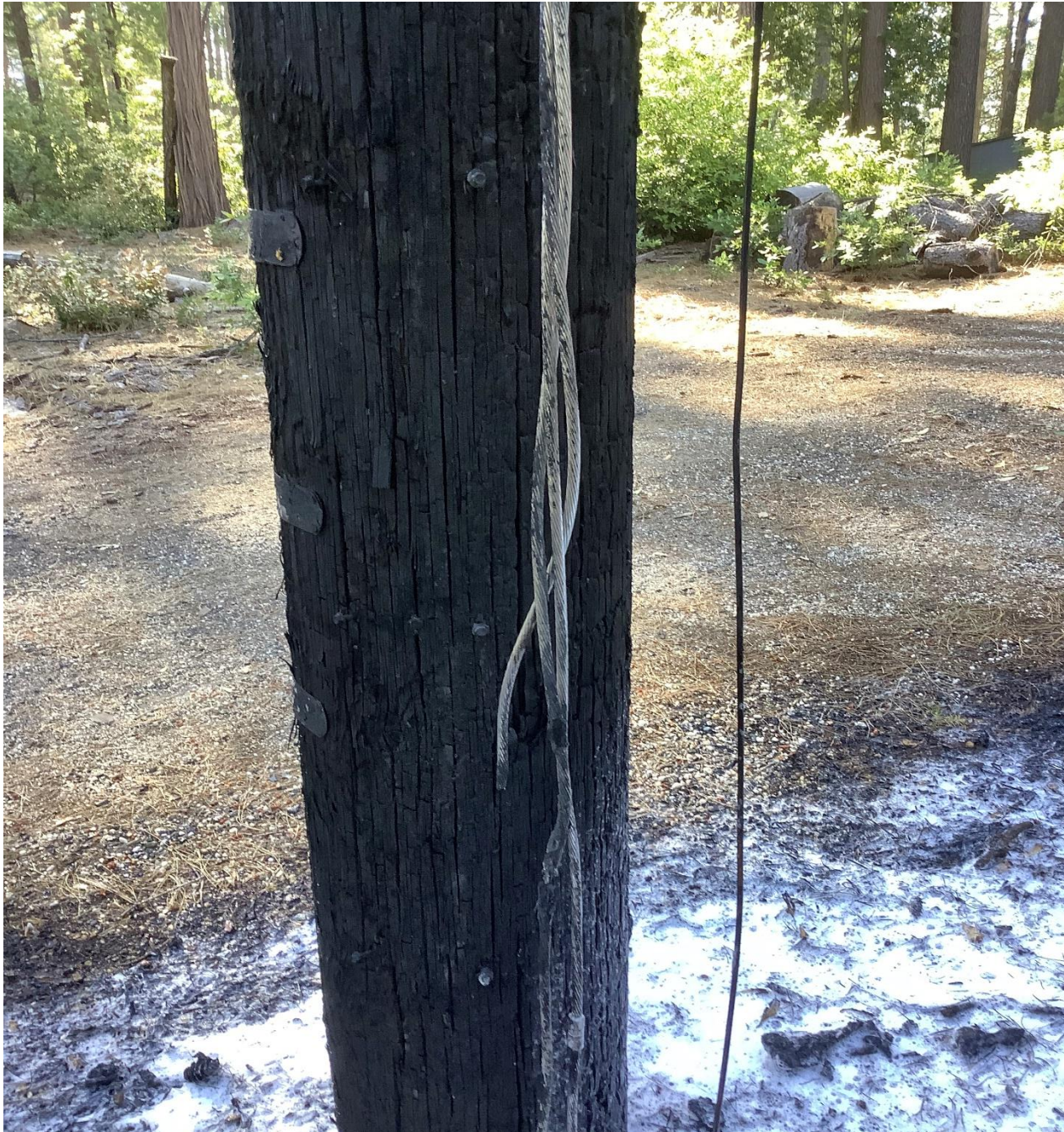
Figure 4 – Ignition and Fire origin area where the secondary riser burnt the molding and service conductor leading to the cause of ignition. Picture taken by the troubleshooter on June 8, 2024.
