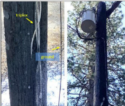
Figure 7 - The pole ignition likely resulted from the failure of a secondary riser involving 1/0 aluminum conductors. A visual inspection of the conductor revealed melting patterns on two hot legs, leading to the breakage of aluminum strands near the ground line.
