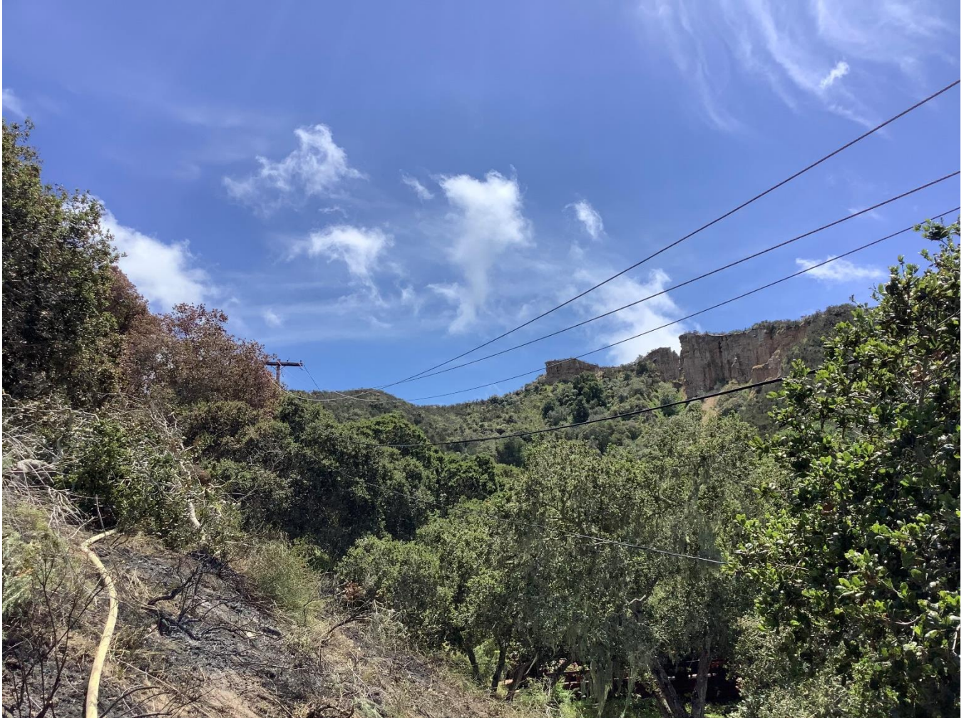
Figure 3 - Fire burn scar area with the Secondary conductors above. Please note, that the tree crew began trimming the vines and branches away from the conductors. Picture taken by the troubleshooter on May 24, 2024
