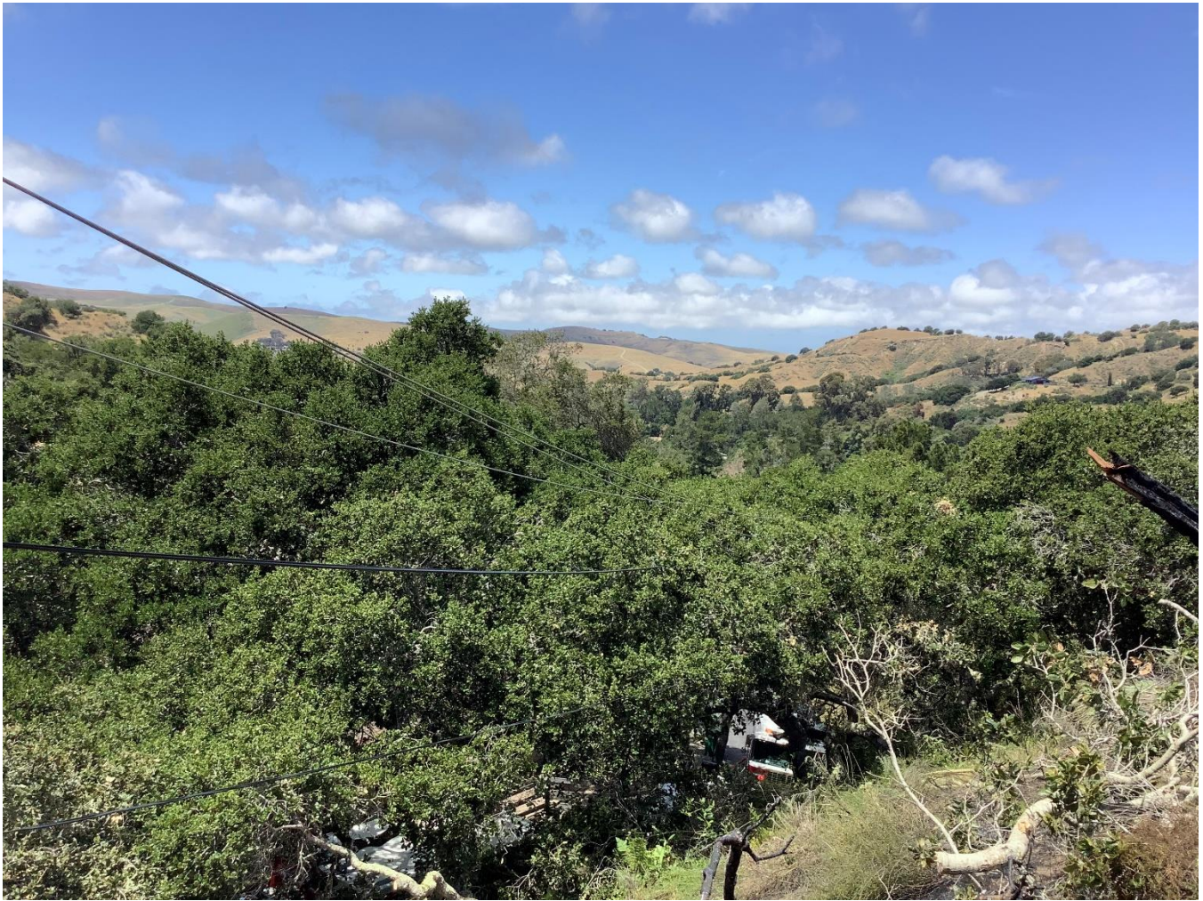
Figure 5 - Secondary conductors going through the trees. Please note, that the tree crew planned on trimming the vines and branches away from the conductors after this picture was taken. Picture taken by the troubleshooter on May 24, 2024
