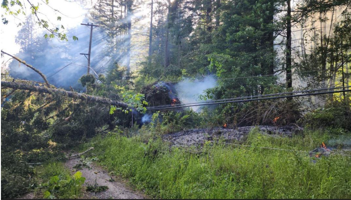
Photo 6: Photo taken by troubleshooter on May 20, 2024 of failed tree taking utility lines down.
