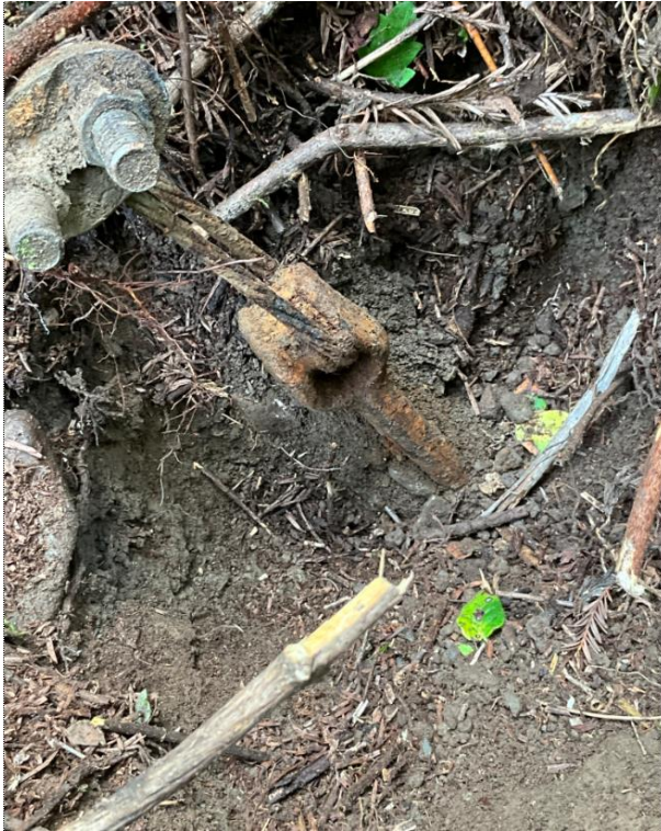
Photo 4: Photo taken by inspector on June 13, 2023, inspection showing damaged anchor.
