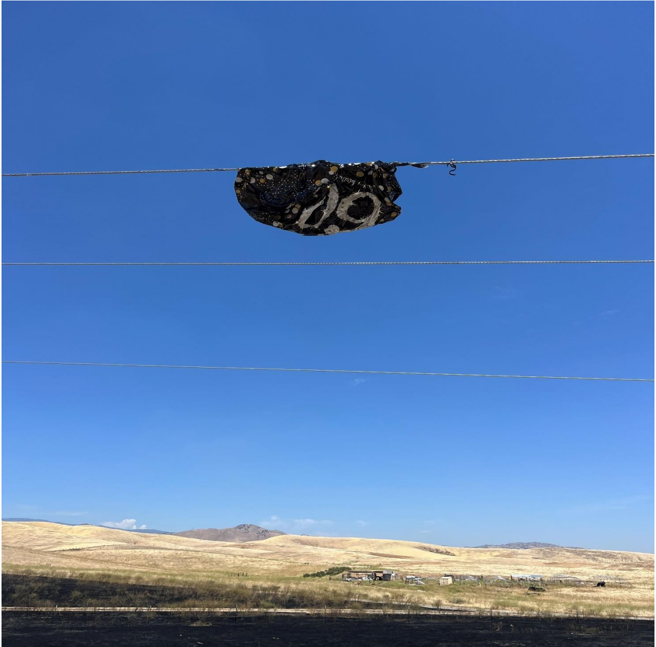
Figure 5 - Mylar balloon remnants found that led to the cause of ignition. Picture taken by the troubleshooter on May 18, 2024.
