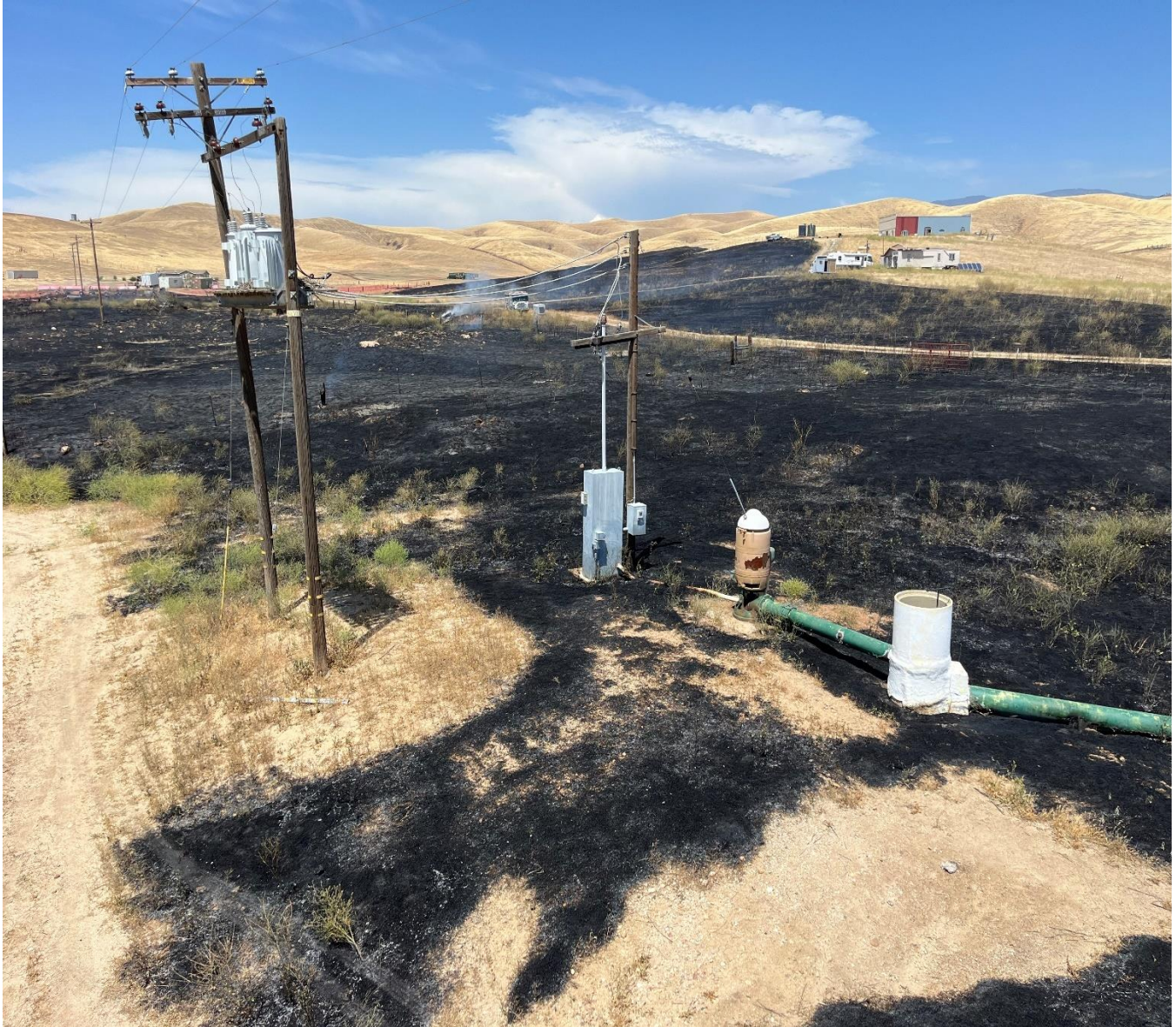
Figure 3 - Fire burn scar area with the mylar balloon remnants found in the conductor above this possible origin location. Please note, that previous pole clearing at this location prevented the fire encroaching our asset SAP Pole ID: 100188521. Picture taken by the troubleshooter on May 18, 2024
