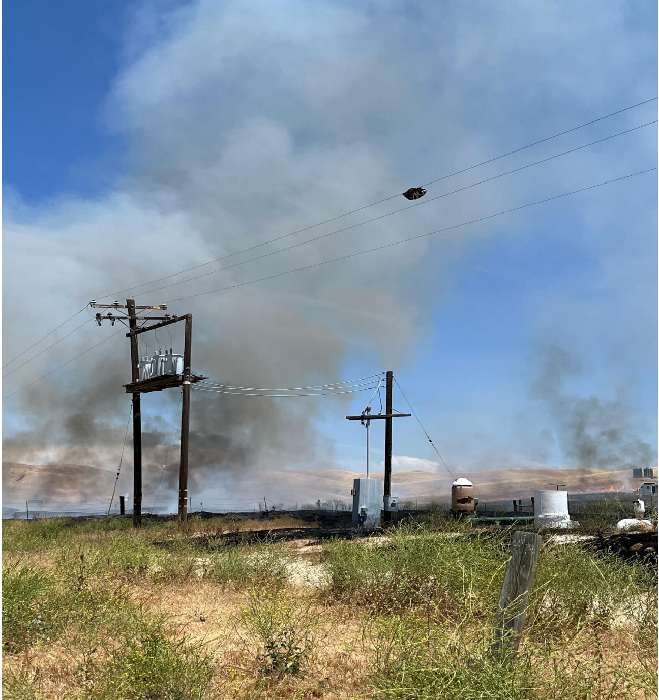
Figure 4 – Ignition and Fire origin area with the mylar balloon remnants found in the conductor that led to the cause of ignition. Picture taken by the troubleshooter on May 18, 2024.
