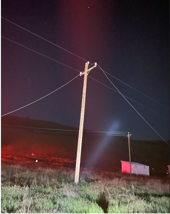
Photo 4 - Photo taken 03/26/24 by troubleshooter showing downed conductor.
