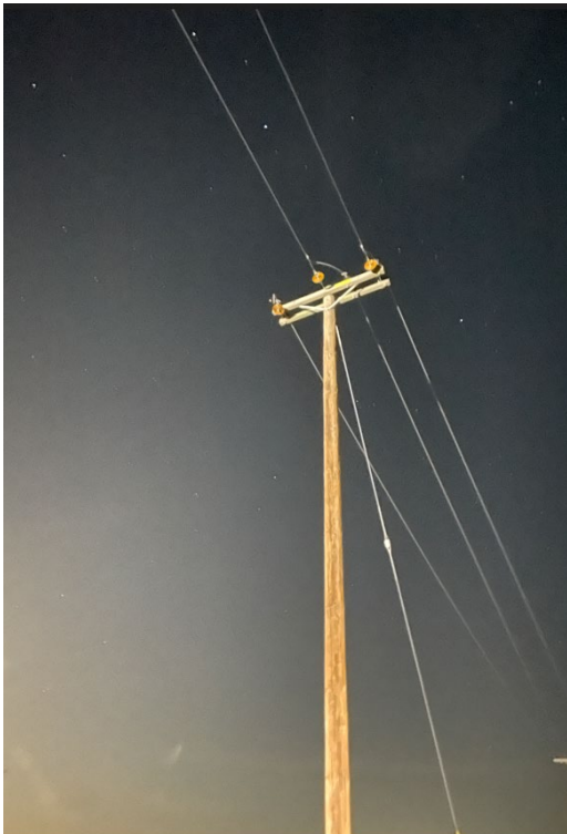
Photo 3- Photo taken 03/26/24 by troubleshooter showing pole top, where conductor broke away.
