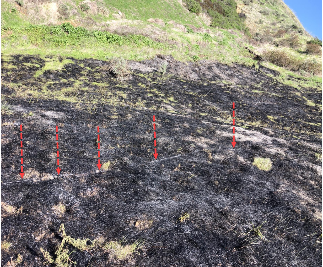
Figure 3 – Part of the burn scar area and one downed conductor phase of the Mesa 1101 12kV distribution circuit. Picture taken by the troubleshooter on February 27, 2024.
