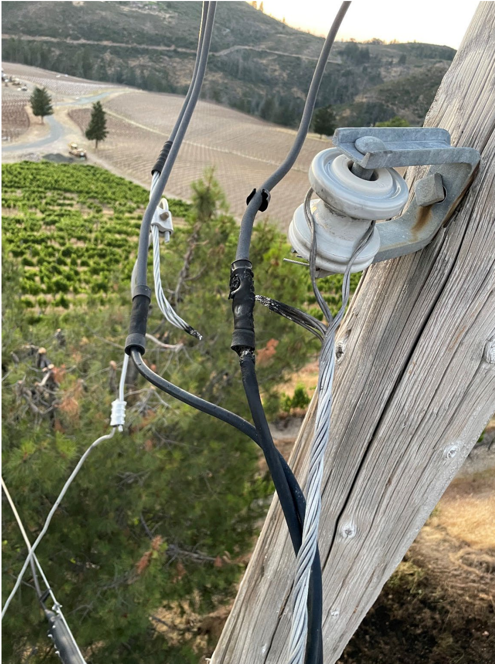
Figure 4 Damaged neutral and hot leg. Photo taken by troubleshooter on June 20, 2024.
