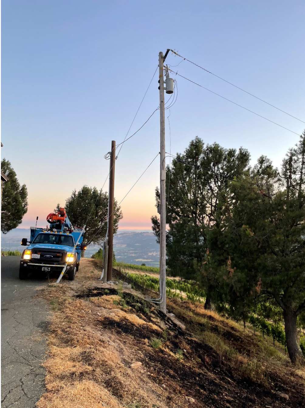
Figure 2 Burn scar at the base of Pole #1, photo facing east. Photo taken by troubleshooter on June 20, 2024.
