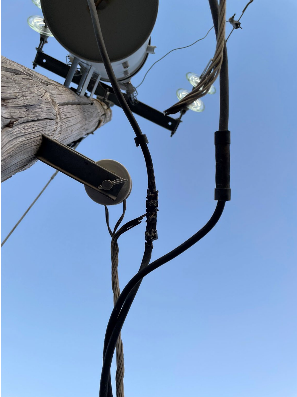
Figure 6 Photo looking up at damaged equipment on Pole #1. Photo taken by troubleshooter on June 20, 2024.
