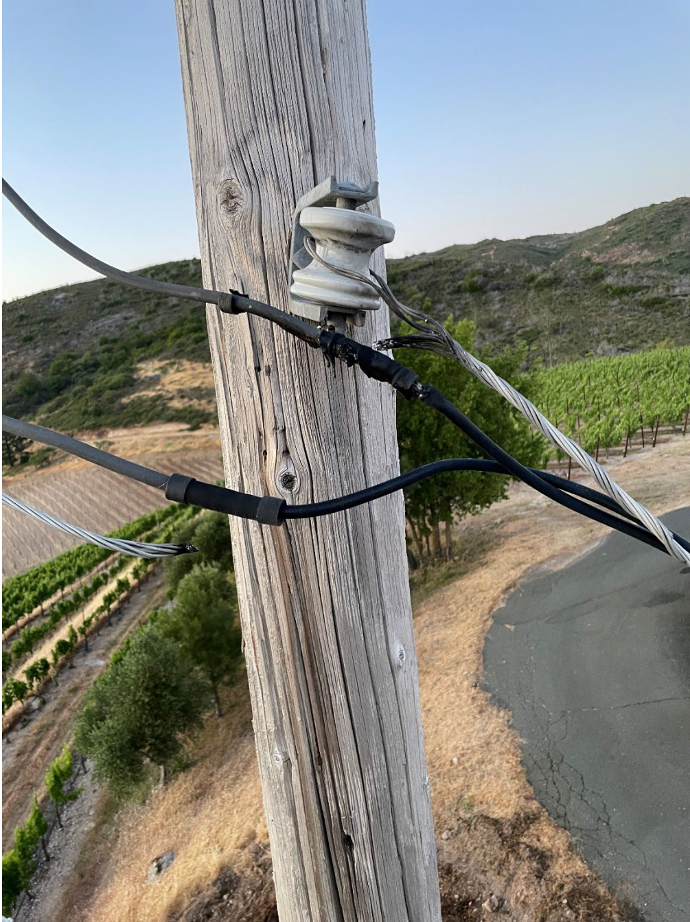
Figure 5 Damaged neutral and hot leg. Photo taken by troubleshooter on June 20, 2024.
