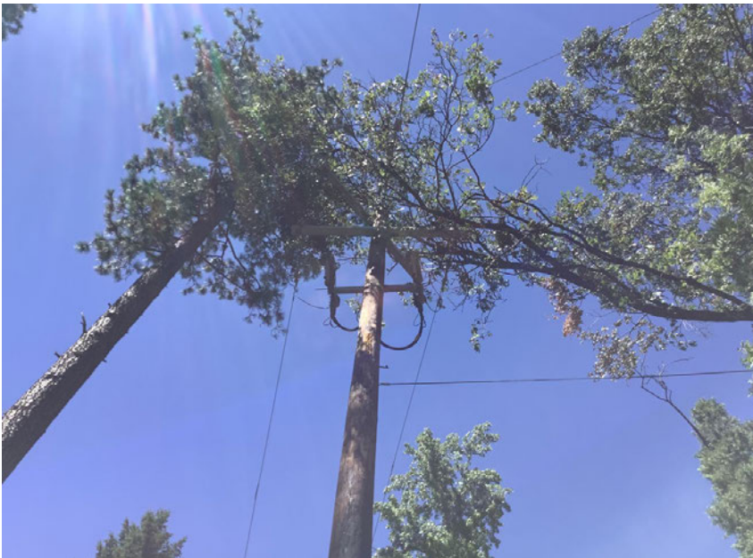
Figure 4 -Troubleshooter photo of failed tree branch on Incident Pole.
