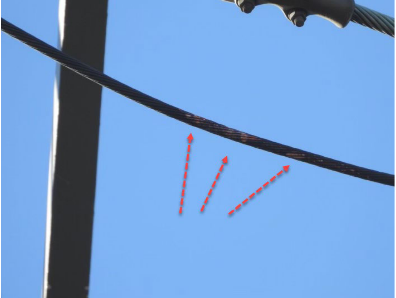
Figure 3 Jumper with arc marks pointed out in the photo. Photo taken by troubleshooter on August 9, 2024.
