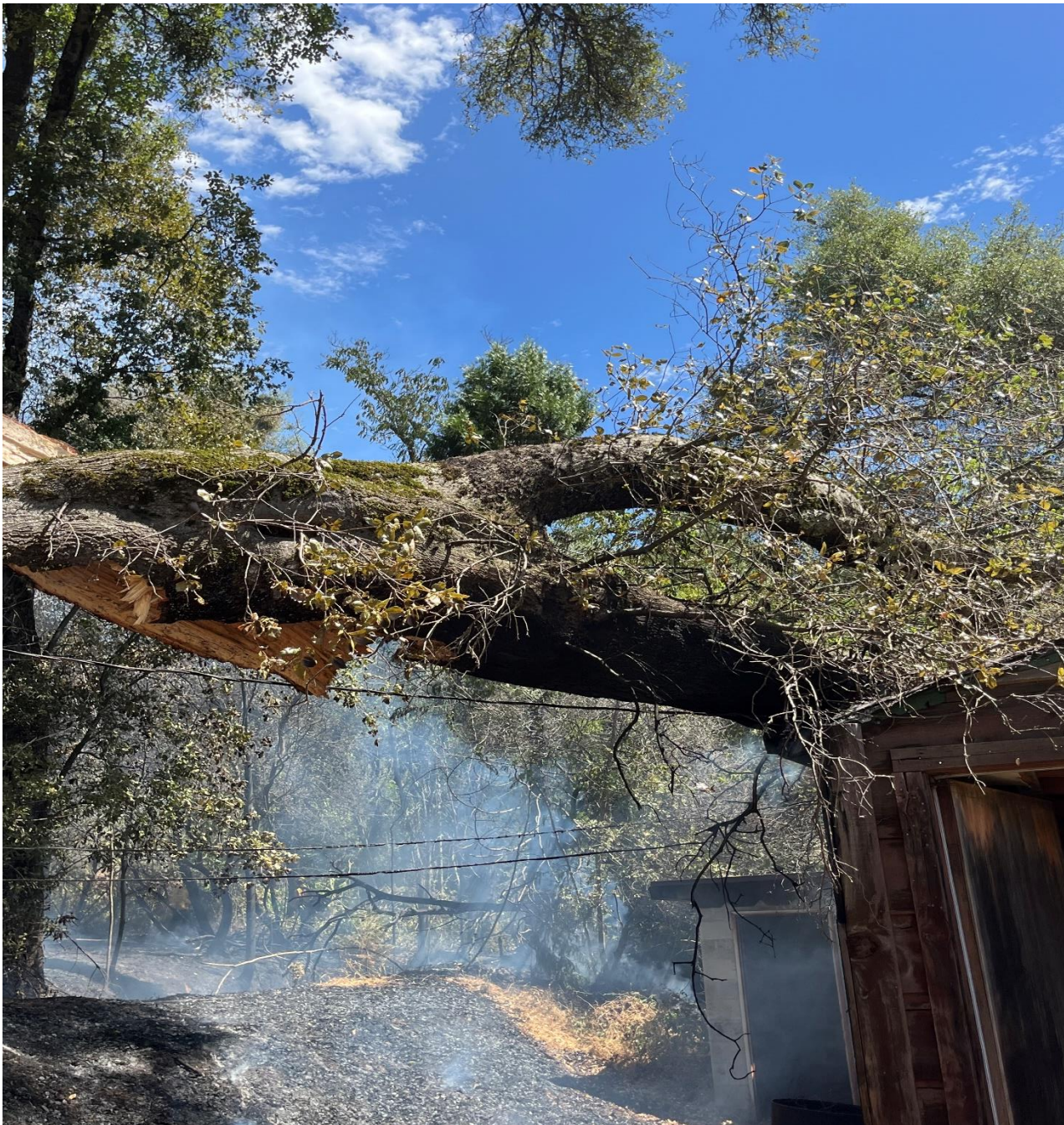
Figure 5 – Close-up of large tree branch/limb fell onto the Secondary Service line conductor which caused arcing and burned vegetation below. Picture taken by the troubleshooter on August 08, 2024.
