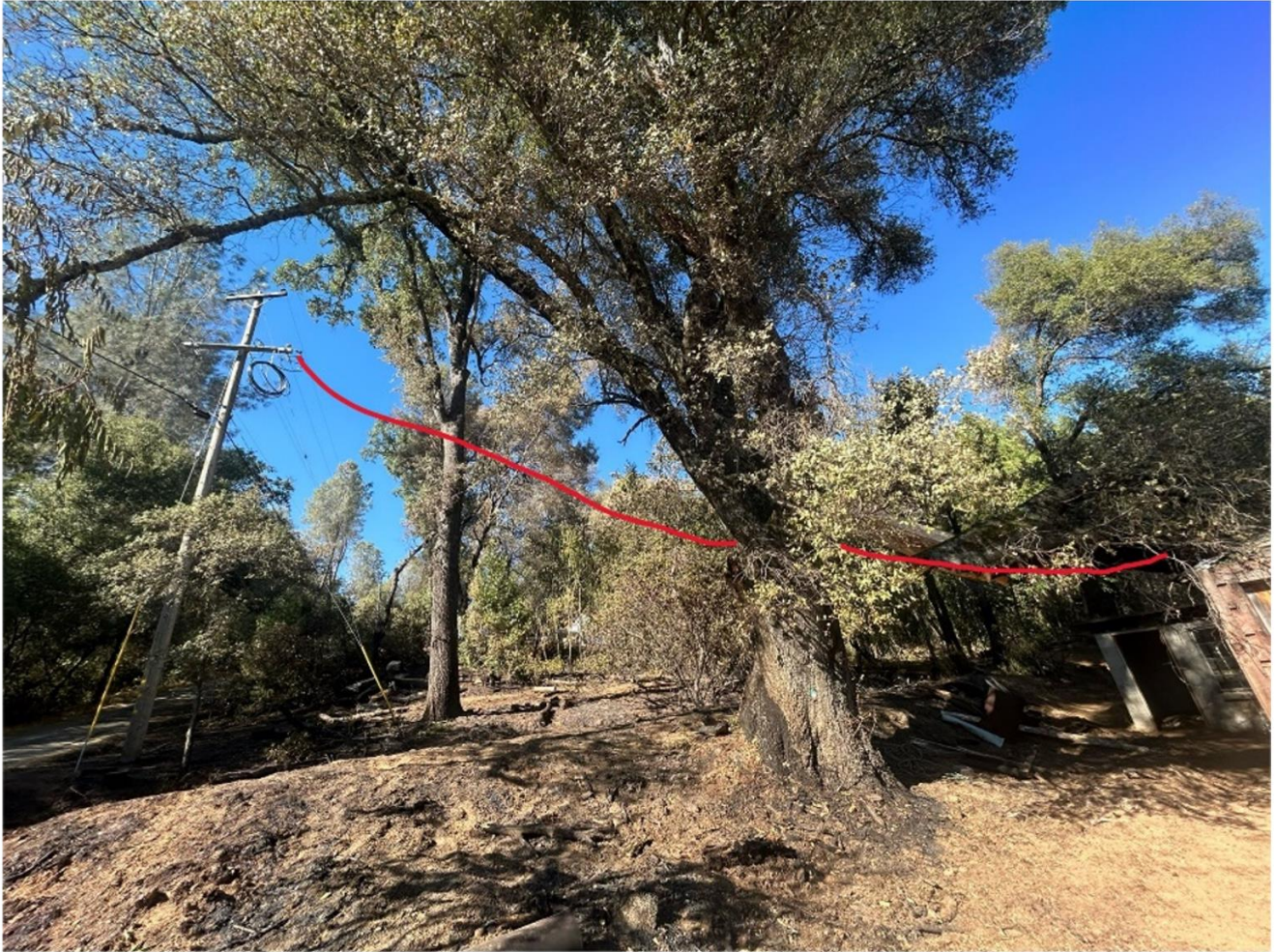
Figure 8 - Service drop detail picture taken by the VM inspector on August 9, 2024.
