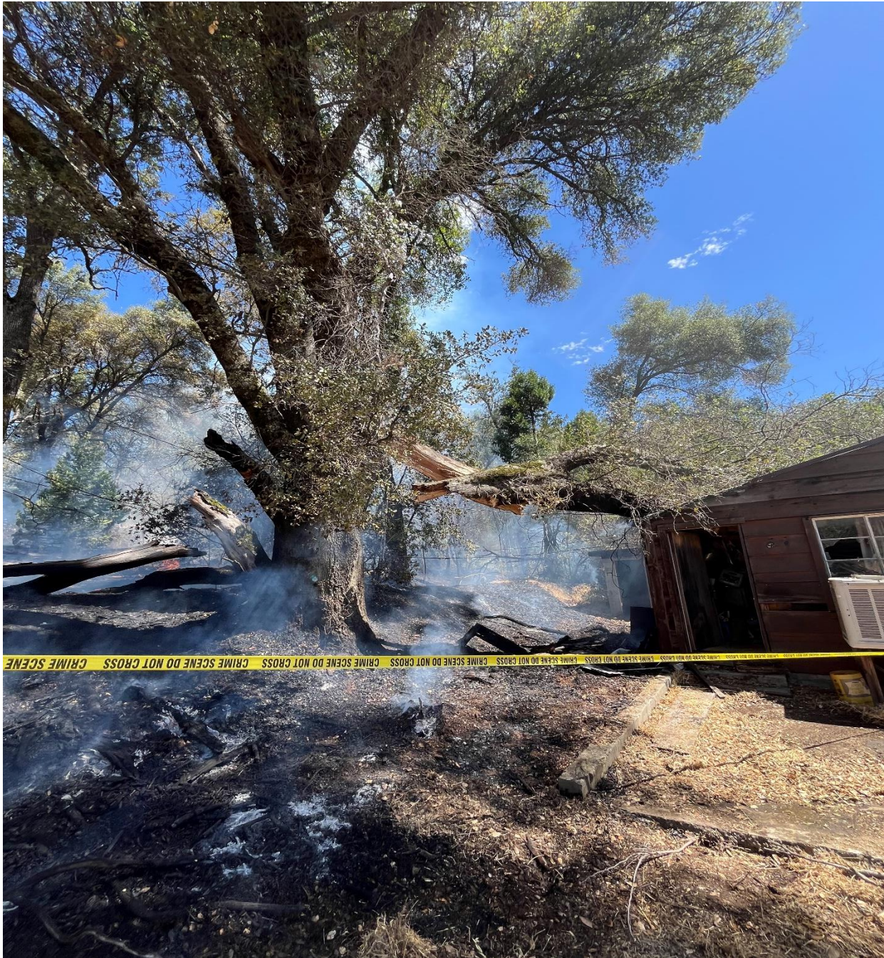
Figure 4 – Ignition and fire origin area where the large tree branch/limb fell onto the Secondary Service line conductor which caused arcing and burned vegetation below. Picture taken by the troubleshooter on August 08, 2024.
