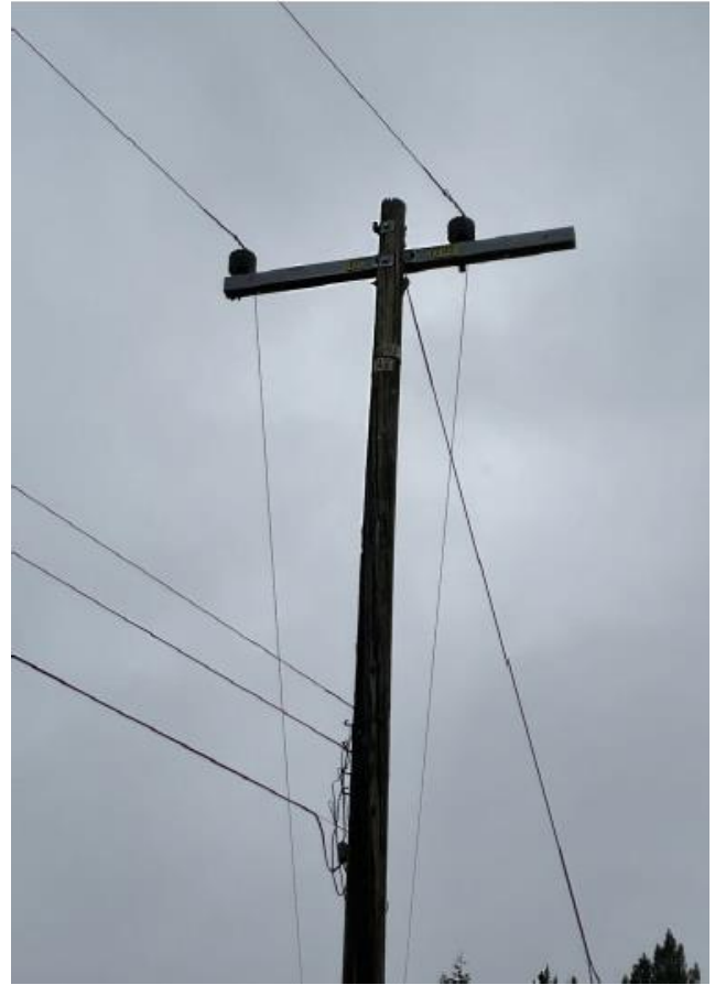
Figure 6 Views of Pole #2 (source side of incident pole) showing crossarm and insulators change between 2019 (left) and 2022 (right). Source: 2019 image: WSIP inspection report # 181-7155634; 2022 image: 2022 GO165 Overhead Inspection report.
