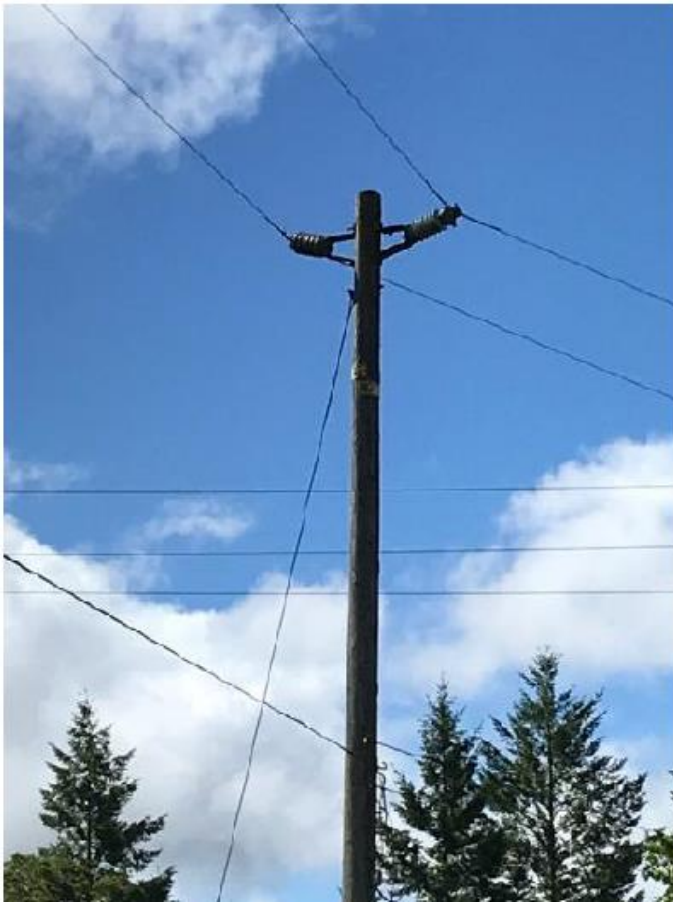
Figure 6 Views of Pole #2 (source side of incident pole) showing crossarm and insulators change between 2019 (left) and 2022 (right). Source: 2019 image: WSIP inspection report # 181-7155634; 2022 image: 2022 GO165 Overhead Inspection report.
