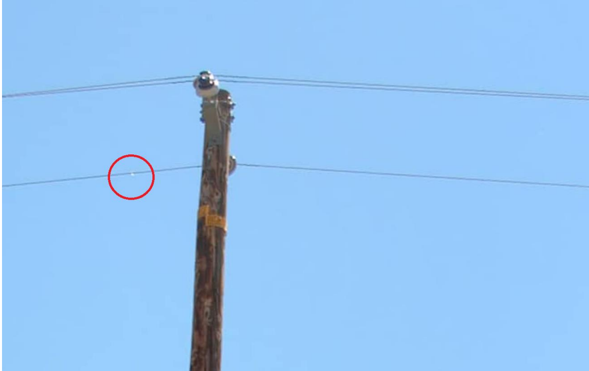
Figure 6. StreetViewer image of pole SAP ID 101510210 from July 8, 2022, showing reflection on conductor. This defect is at the same approximate location on the same span where the conductor broke in this incident.
