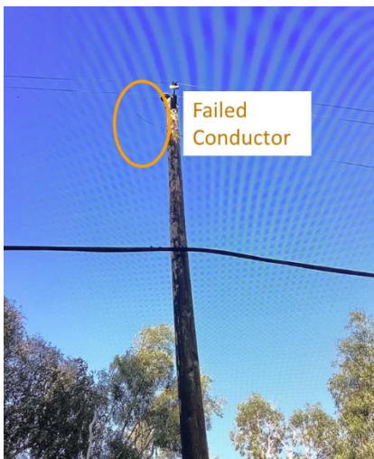
Figure 3. Incident photos taken July 9, 2024 showing failed conductor from Pole SAP ID 101510120 (left), failed conductor on ground (center), and burn area around pole (right).
