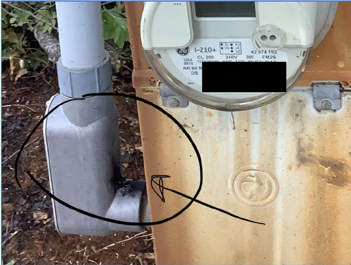
Figure 4 Photo by Troubleman on July 6, 2024 indicating observed arcing marks next to the meter panel.
