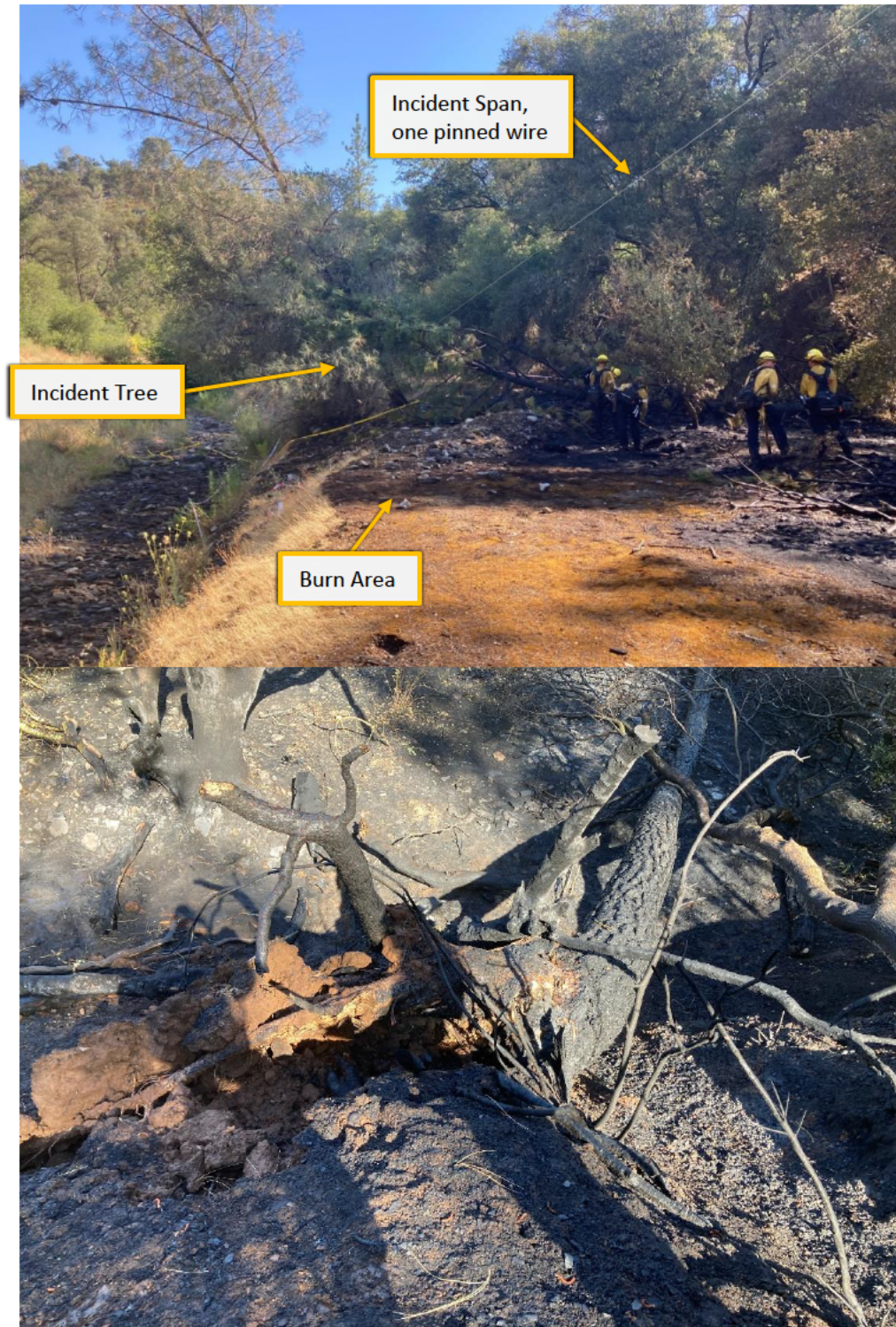
Figure 7. Photos of fallen tree on Incident Span (top) and close-up of tree roots (bottom) (Vegetation Management, taken July 6, 2024).
