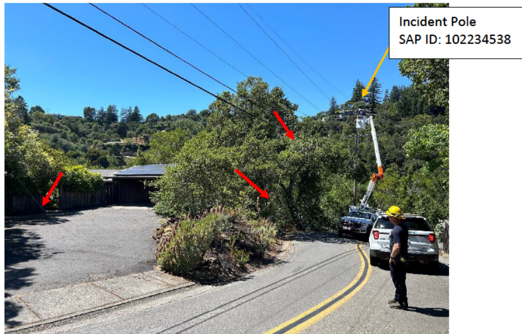
Figure 5 Views of burnt vegetation caused by downed Incident Conductor and downed wire (red arrows in bottom photograph indicate location). Source: Troubleshooters images taken on July 5, 2024.
