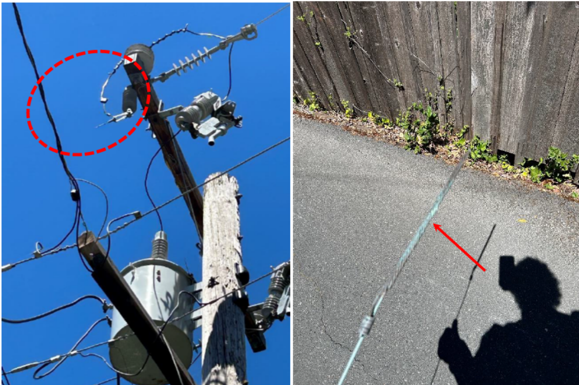
Figure 6 Location where Incident Conductor broke at Pole 2 prior to the incident (top, source Google Maps, February 2023) and after the incident (bottom, Source: EC # 129175534). The failure location is indicated with a circle and the tap guard is indicated with arrows in the photographs.
