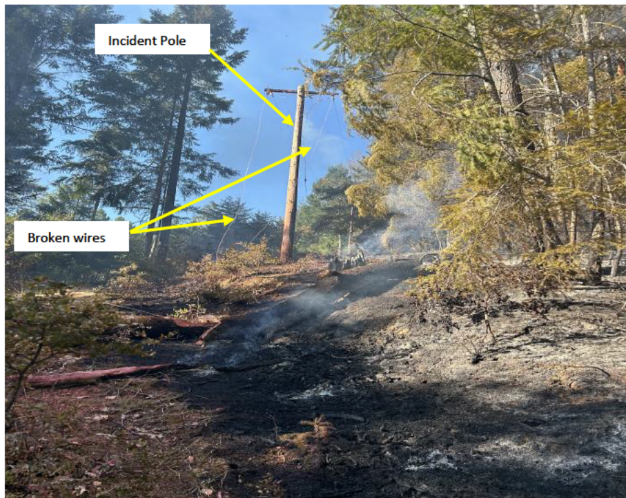
Figure 4 Photograph showing broken wires, Incident Pole, fallen trunk and smouldering vegetation. Photograph Source: EC# 129175992 (dated July 5, 2024)
