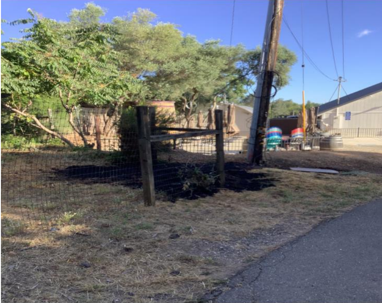
Figure 2 SAP Pole ID 100045817 with burn scar at the base of the pole. Photo taken by troubleshooter on June 27, 2024.
