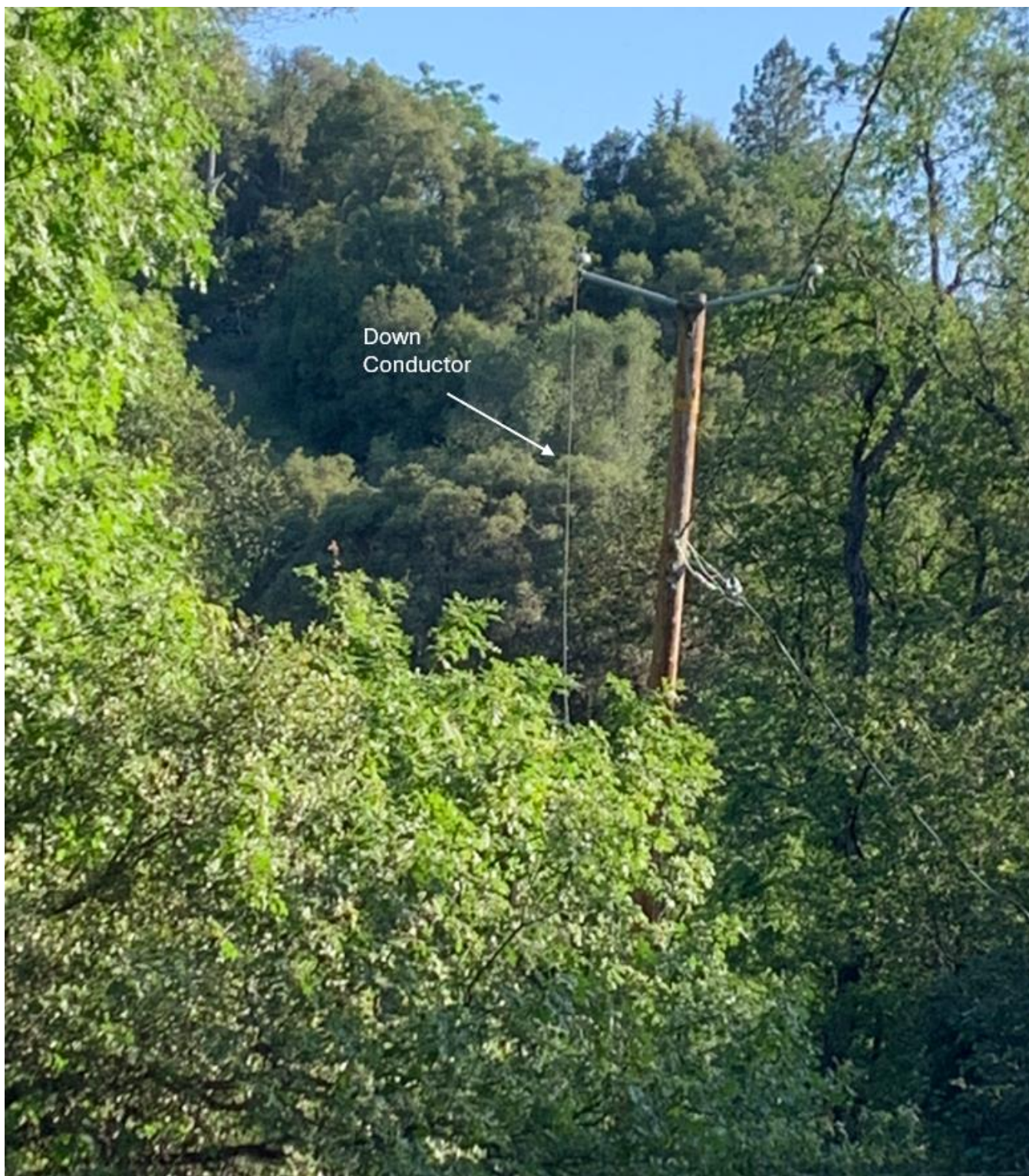
Figure 5 Photo depicting south phase down conductor on SAP ID # 101050282 taken by troubleshooter.
