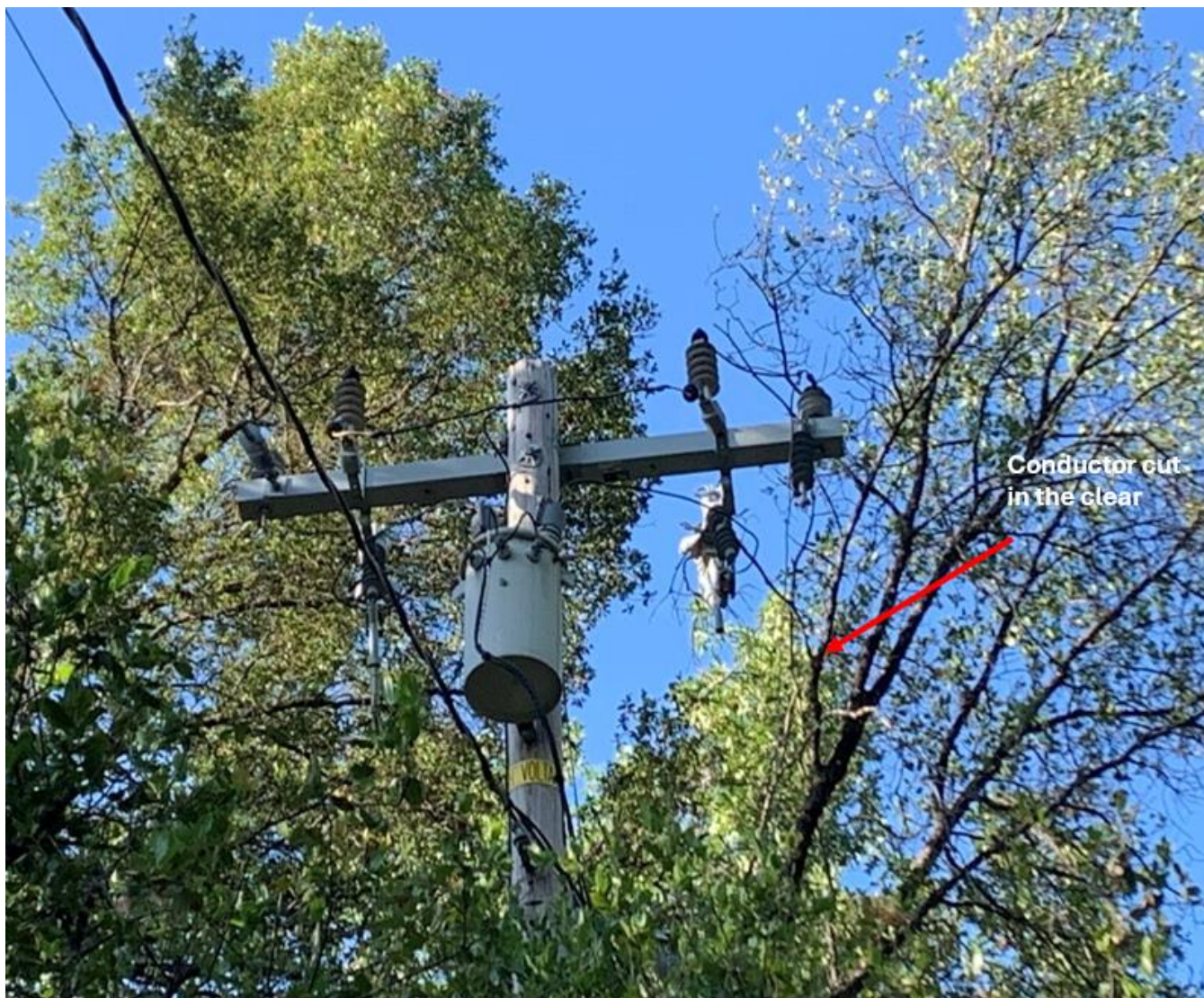
Figure 4 Photo depicting south phase conductor cut in the clear near SAP Id #101050291 taken by troubleshooter.
