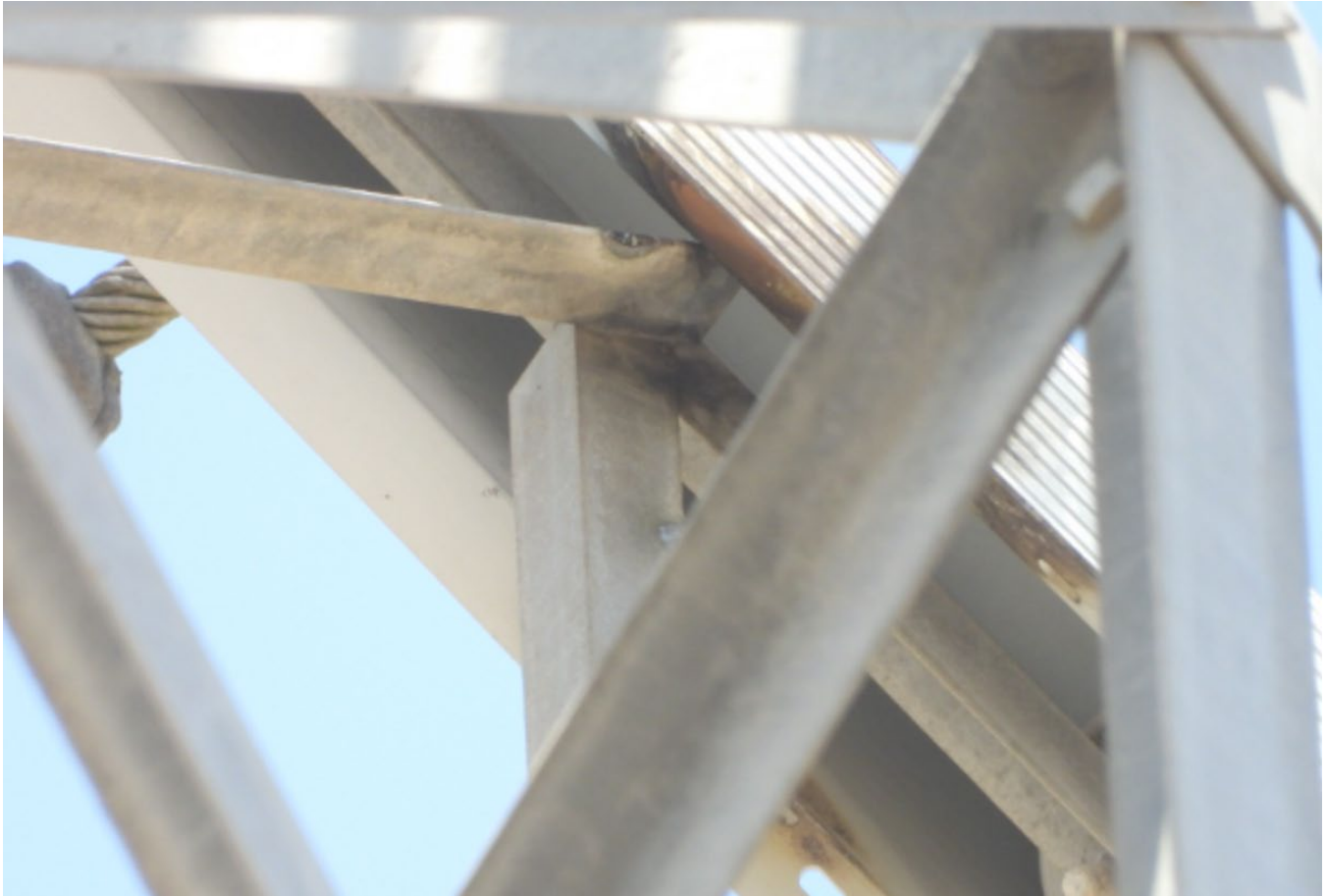
Figure 8 – Photo of arc on bird guard and structure.
