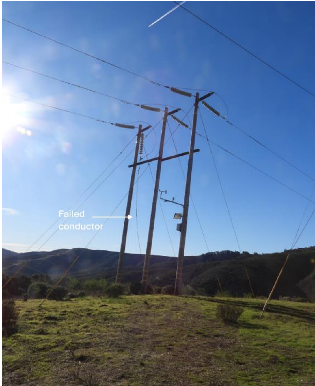
Figure 3 Photo of three-pole transmission structure where failed conductor occurred taken by troubleshooter on date of incident.
