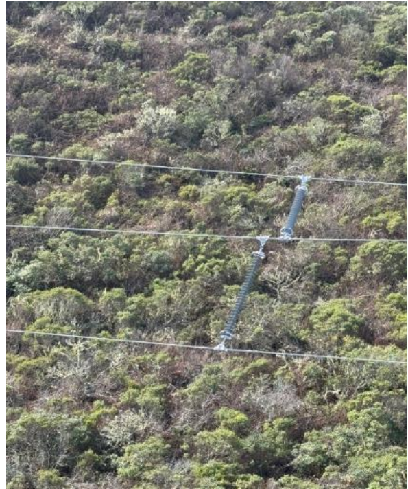
Figure 8 & 9 Photos from LC Notification 129928954 showing spacers that were installed between poles ?01/13 and ?02/0 to temporarily mitigate conductor midspan on December 16, 2024.
