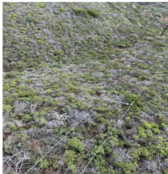
Figure 10 & 11 Photos from LC Notification 129928956 showing spacers that were installed between poles ?4/0 and ?4/1 to temporarily mitigate conductor midspan on December 16, 2024.
