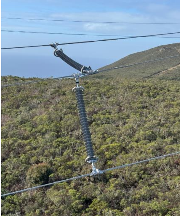
Figure 8 & 9 Photos from LC Notification 129928954 showing spacers that were installed between poles ?01/13 and ?02/0 to temporarily mitigate conductor midspan on December 16, 2024.
