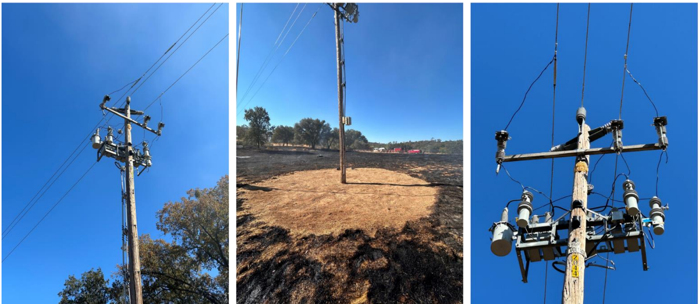
Figure 3. Incident photos showing pole SAP ID 101380976 (left), burned area outside of base of pole (center), and capacitor bank C2044 (right) (taken October 14, 2024).
