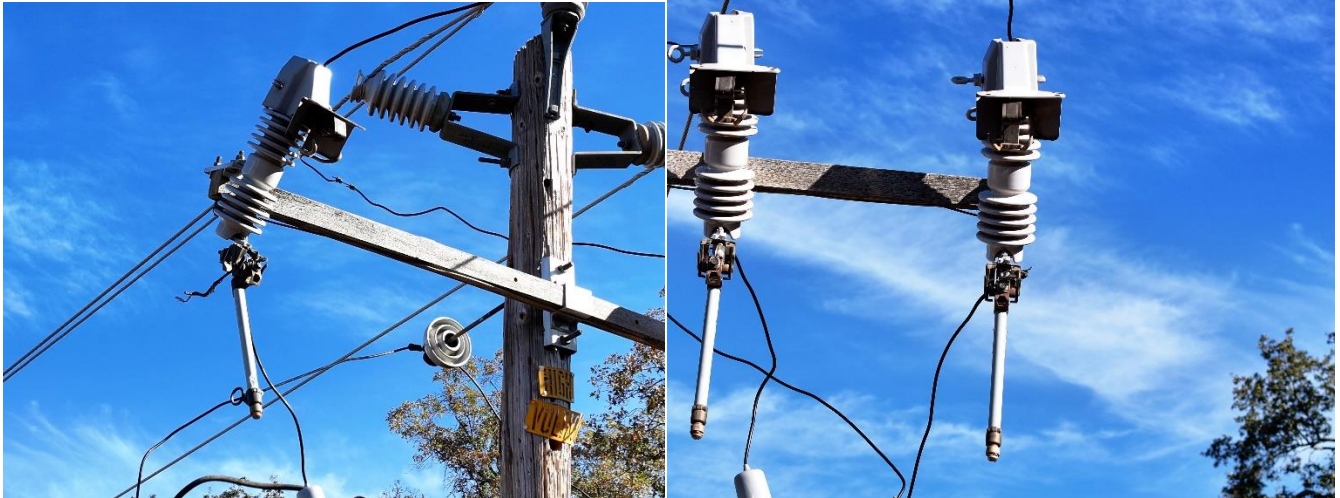
Figure 6. Post-incident photos showing blown fuses on capacitor bank C2044 (taken October 22, 2024).
