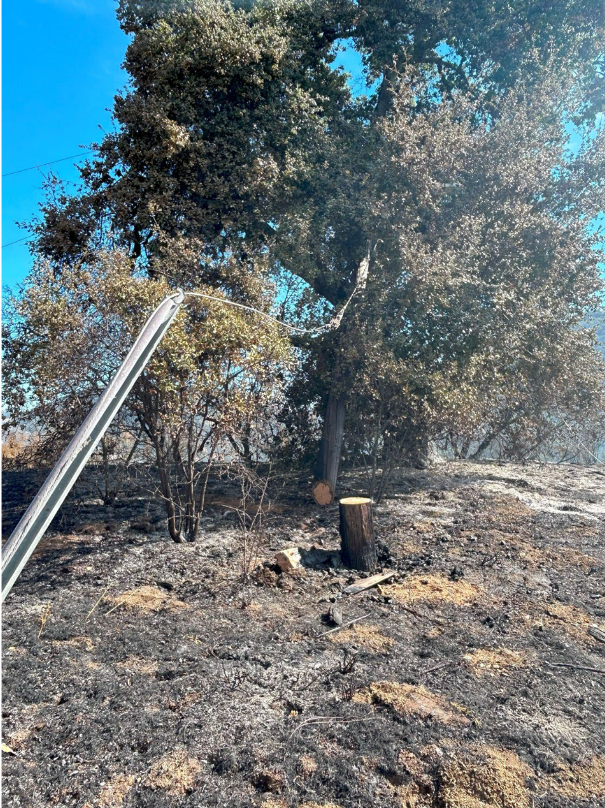
Figure 13: Burned/broken Pole #2 (SAPID 101702582 ) at top of hill; photo taken by ignitions investigator October 9, 2024
