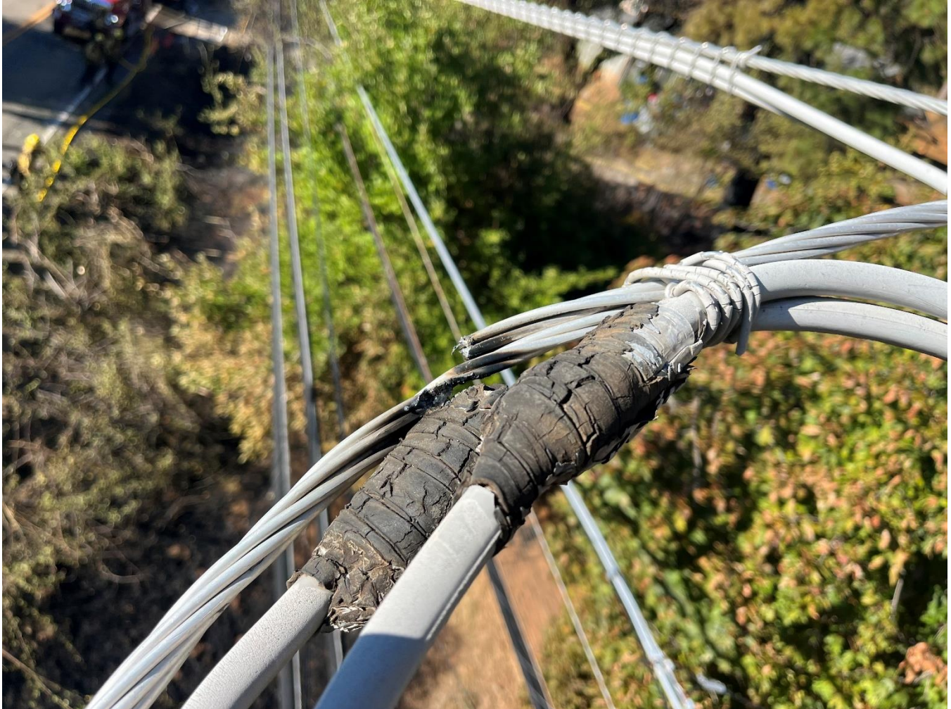
Figure 3. Incident photo showing damaged grey AWAC conductor and service conductor.
