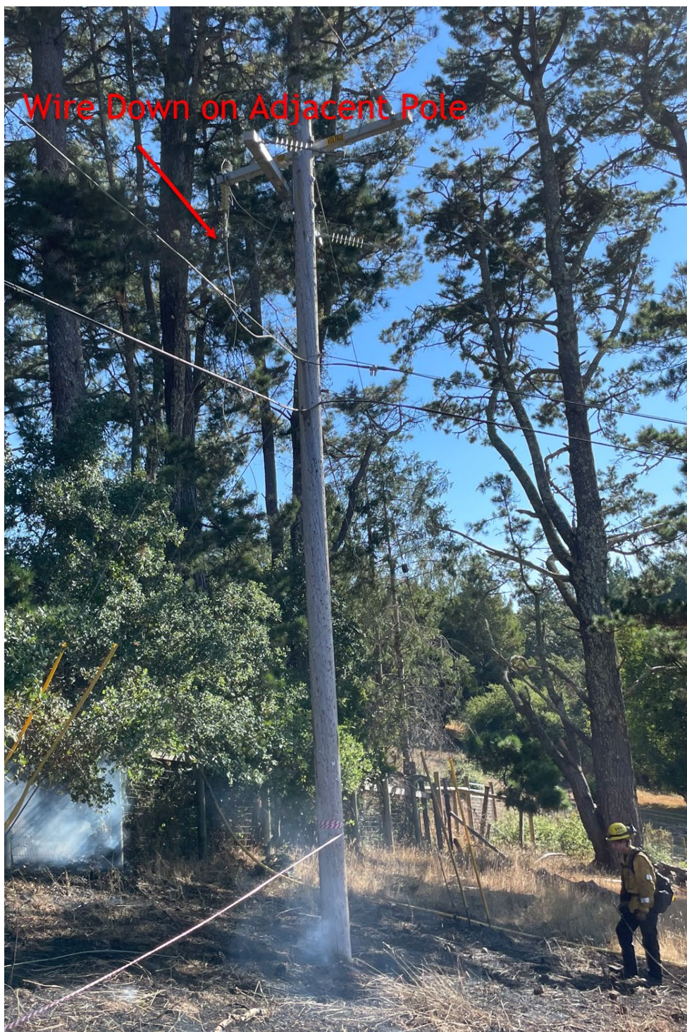
Figure 2 – Wire down on adjacent pole SAP ID 102009312 on August 25, 2024. Photo taken by the troubleshooter.
