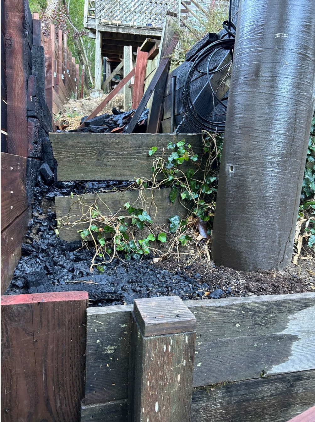
Figure 2 Burn scar at the base of pole. Photo taken by troubleshooter on August 16, 2024
