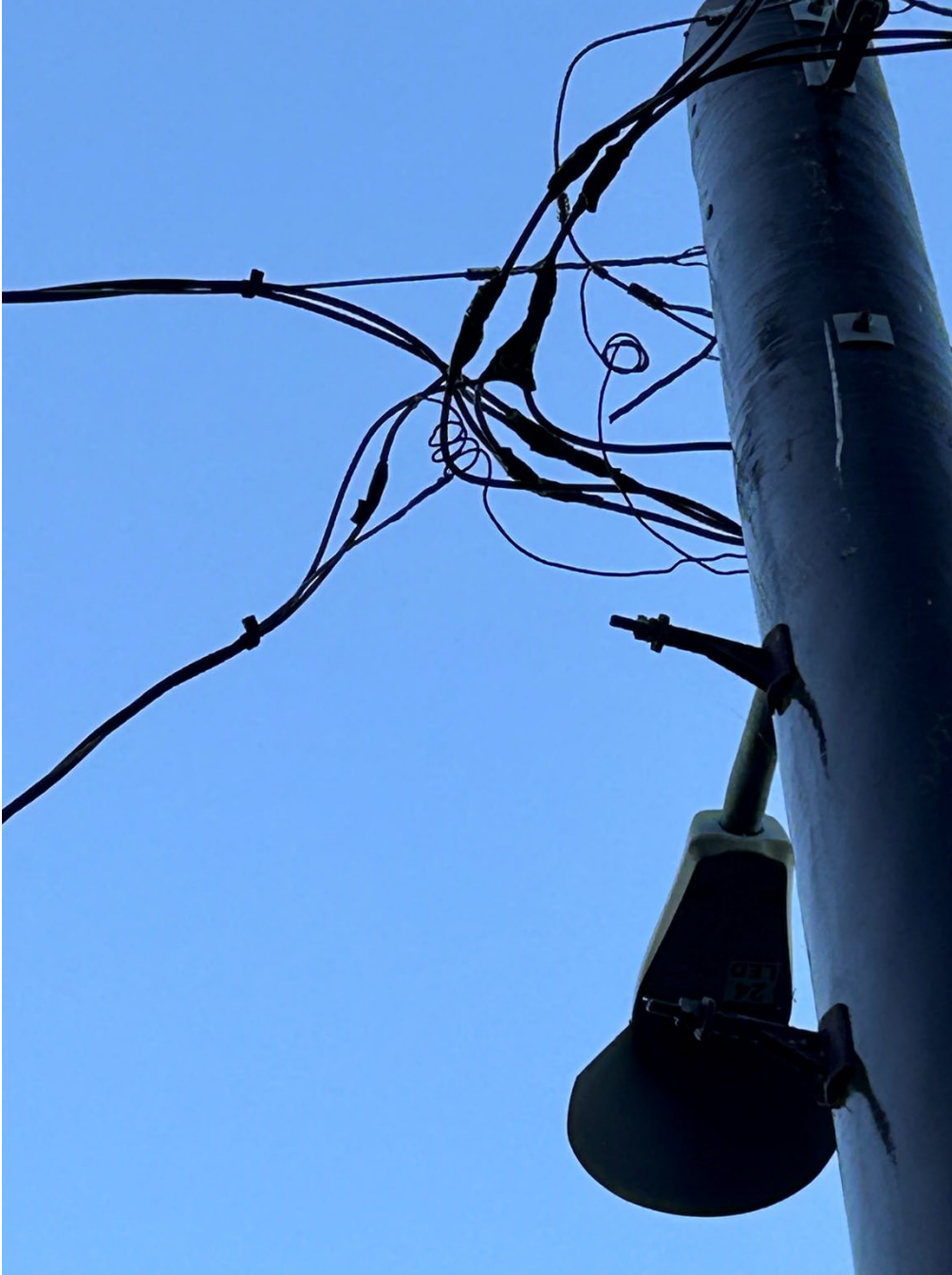
Figure 5 Damaged neutral and hot leg. Photo taken by troubleshooter on August 16, 2024
