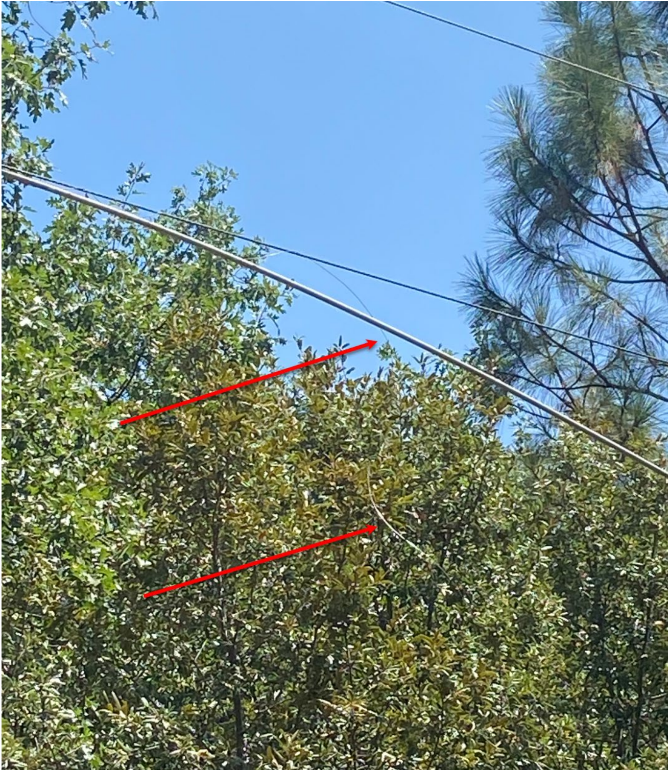
Figure 2 – View of broken tie wire on the phone cables on July 29, 2024. Photo taken by the troubleshooter.
