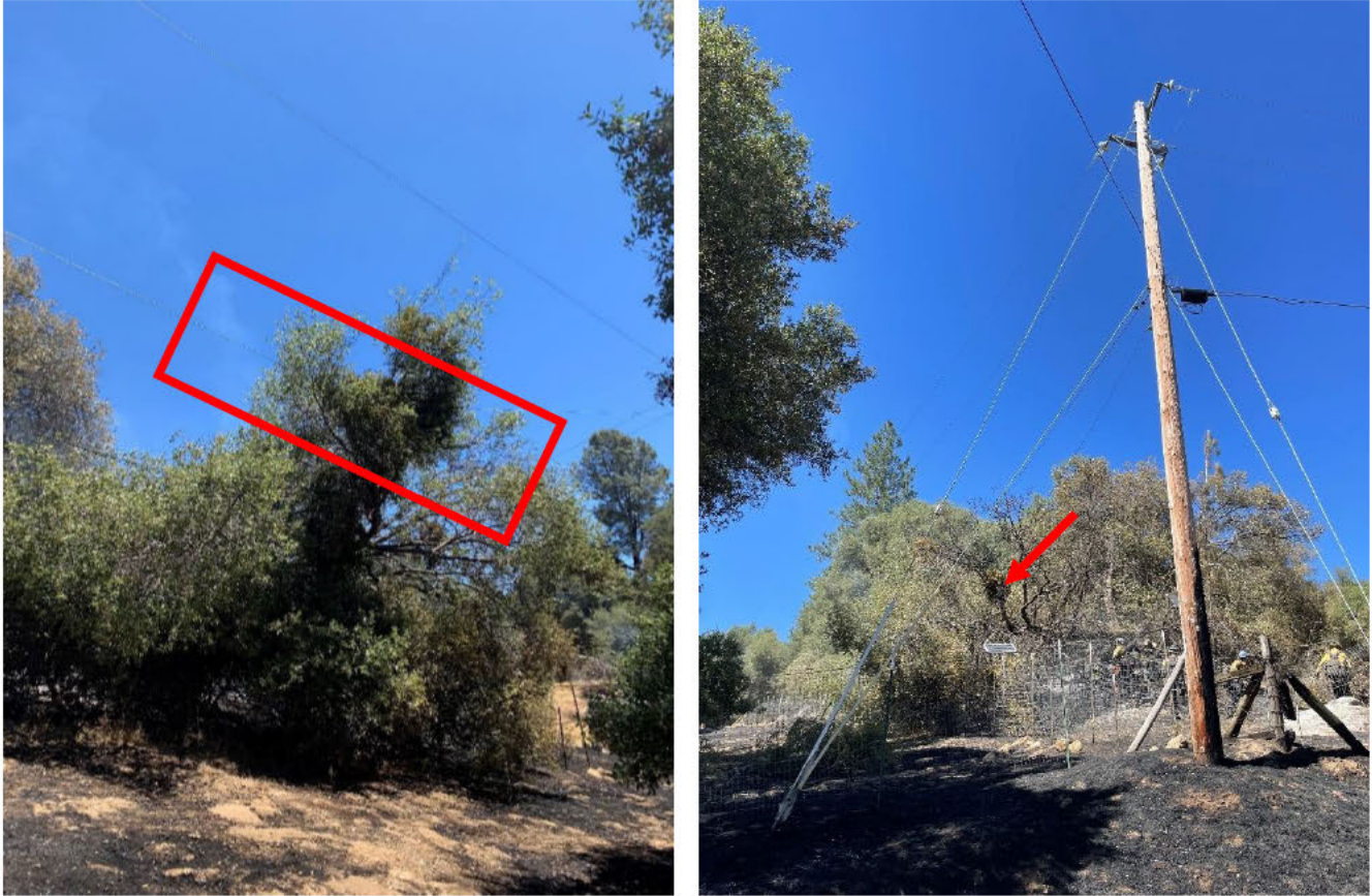
Figure 2. Photograph taken at approximately 1340 hours depicting the Incident Tree branch in contact with the east phase (left, indicated, looking east), and photograph taken at approximately 1505 hours after the Incident Tree (right, looking north) had been removed by the troubleshooter.
