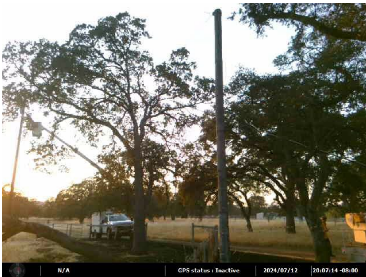
Figure 3 – View of the Incident Pole with failed tree limb also shown on the ground on July 12, 2024. Photo taken by the troubleshooter.
