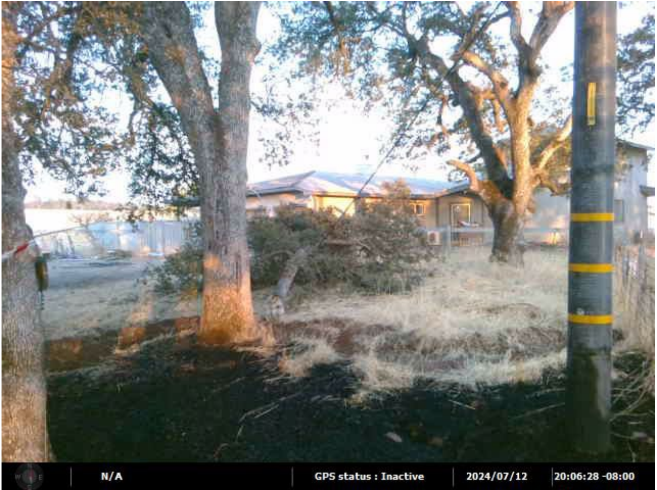
Figure 2 – View of failed tree limb into the secondary with a portion of the burn scar shown near the Incident Pole on July 12, 2024. Photo taken by the troubleshooter.
