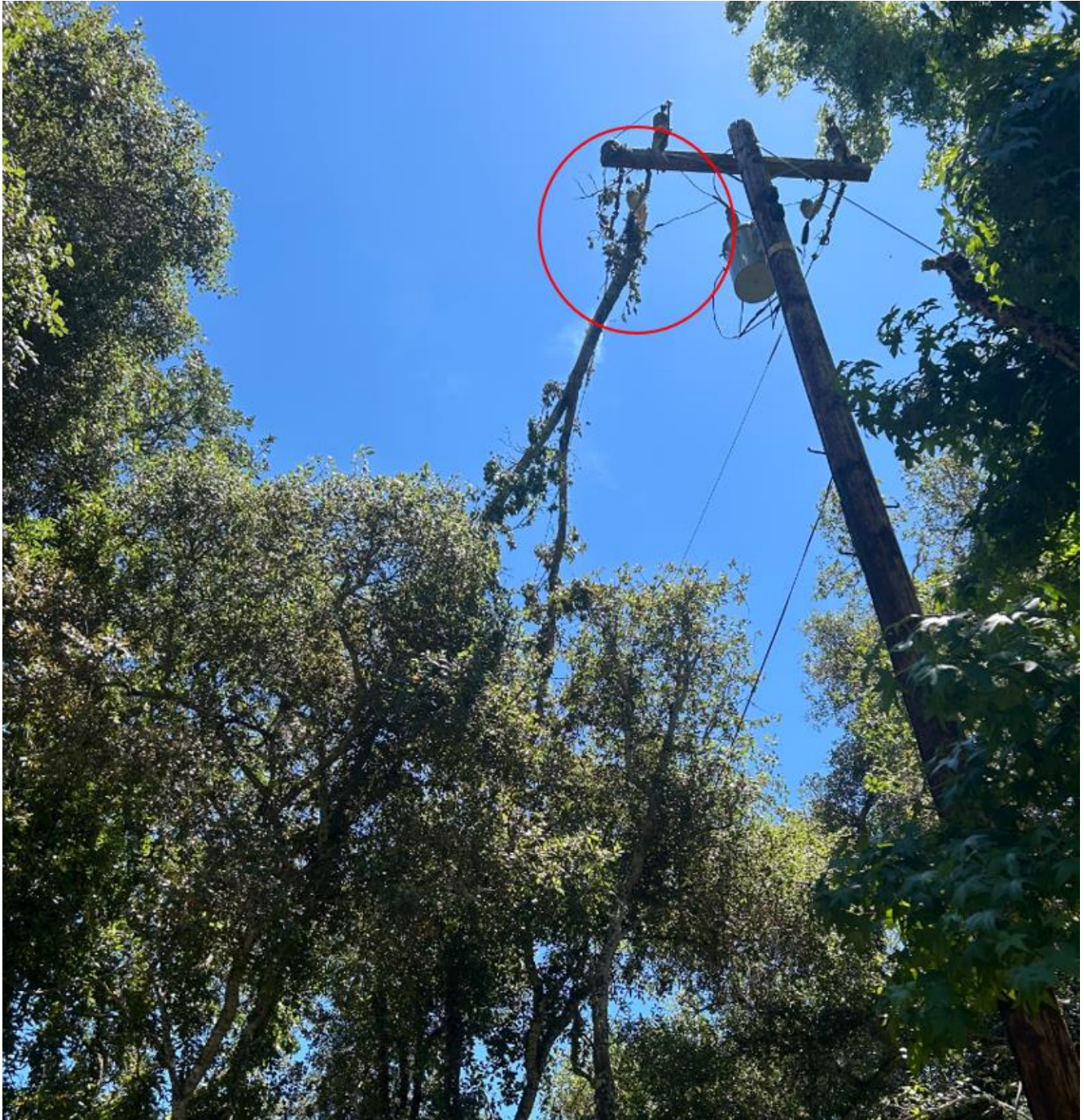
Figure 3 Photo depicts fallen branch (circled in red) on overhead conductor near pole SAP ID # 102212964 taken by troubleshooter on July 3, 2024.
