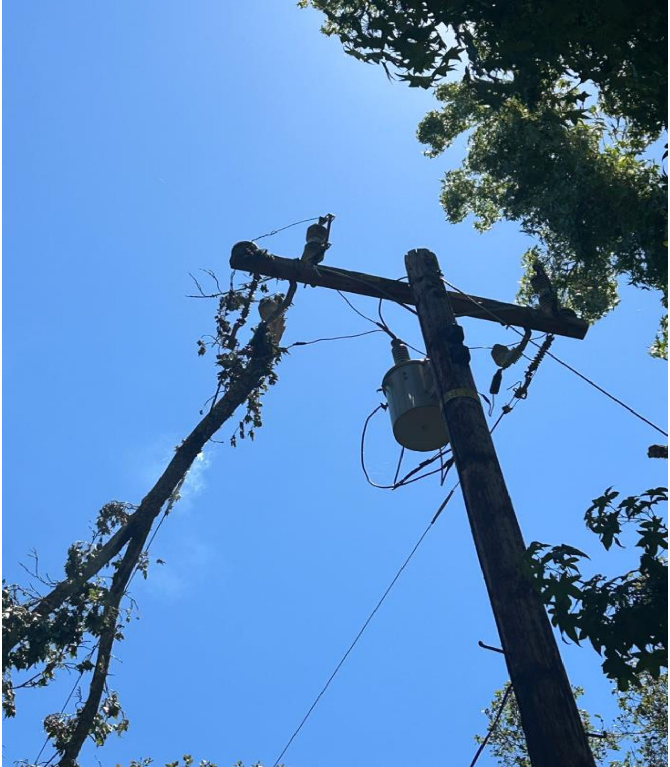
Figure 4 Close up photo of fallen branch on overhead conductor taken by troubleshooter on July 3, 2024.
