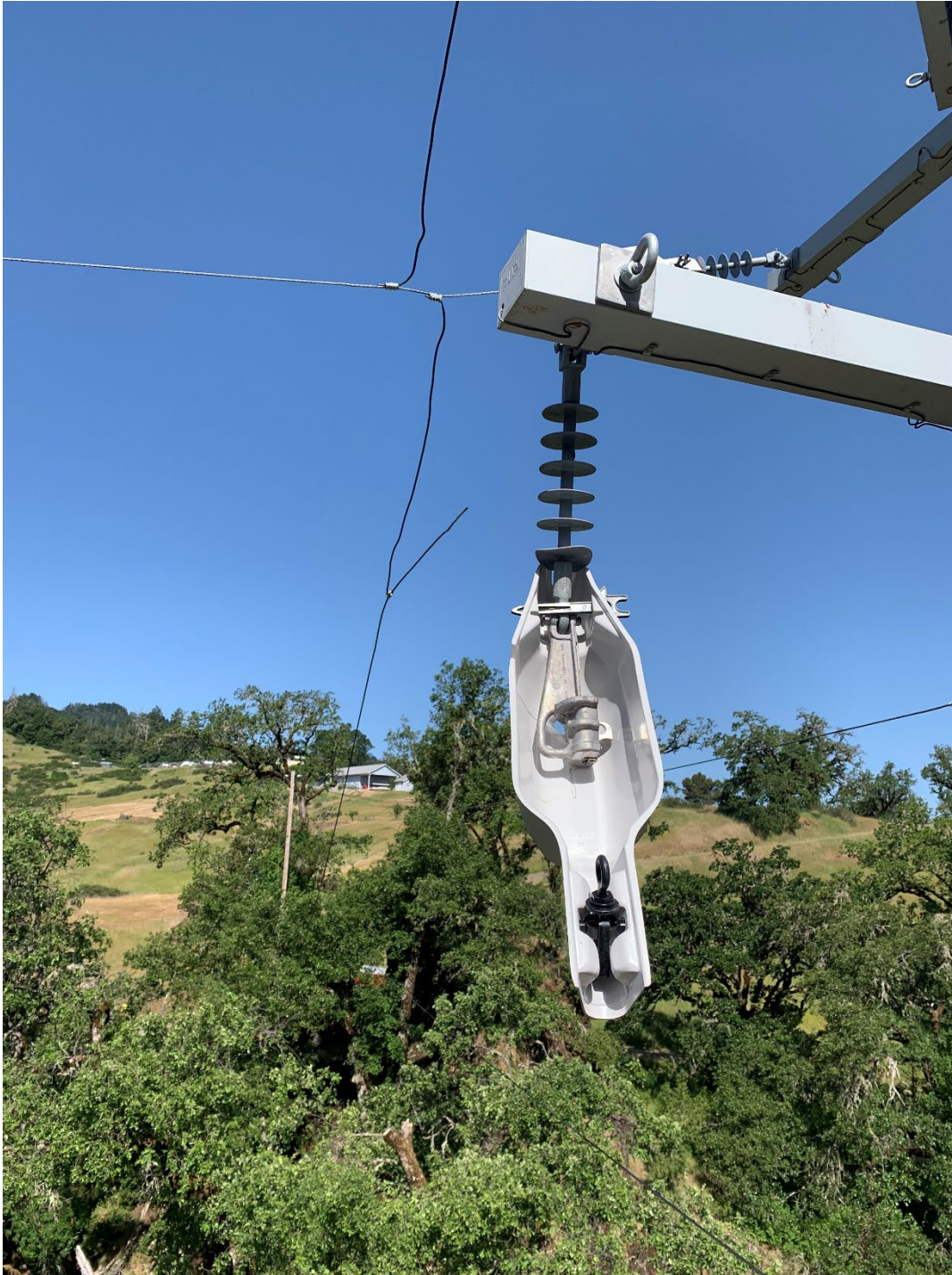
Figure 4 – Incident span shown with wire detached from dead-end shoe. Photo taken by the troubleshooter.
