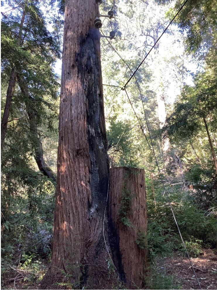
Figure 4 – Photo of tree connect SAP ID 103493985 and fire damage. Photo taken by the troubleshooter.
