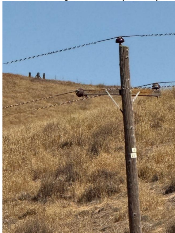
Figure 20: Wind related damage in Monterey County – Broken crossarm
