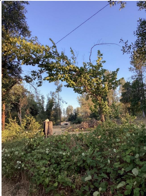
Figure 18: Vegetation hazard in Shasta County –Tree fell on service line
