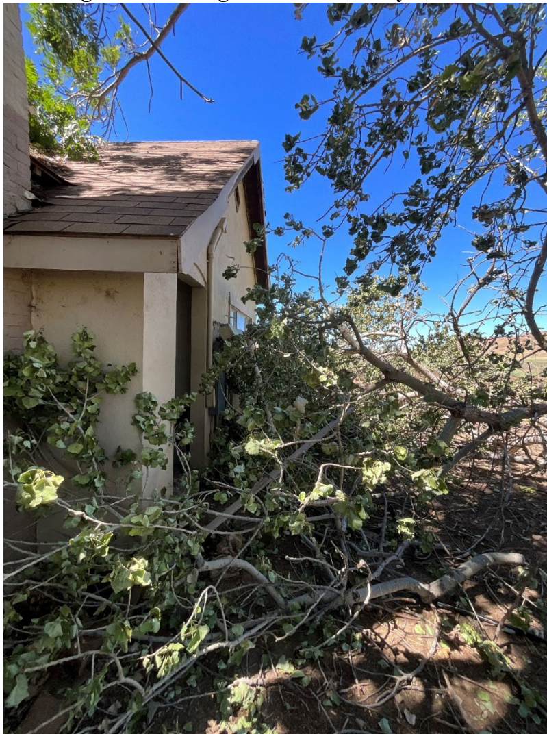
Figure 18: Vegetation Damage in Colusa County – Broken Conductor
