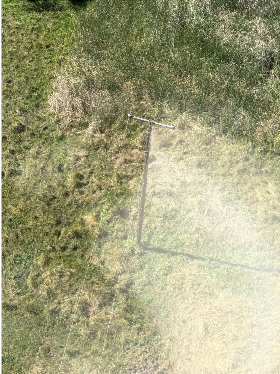
Figure 21: Wind Damage in Glenn County – Broken Tie Wire
