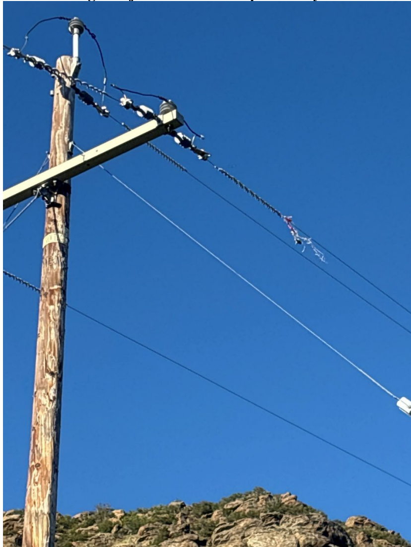
Figure 18: Foreign Object Hazard in Napa County – Balloon on line
