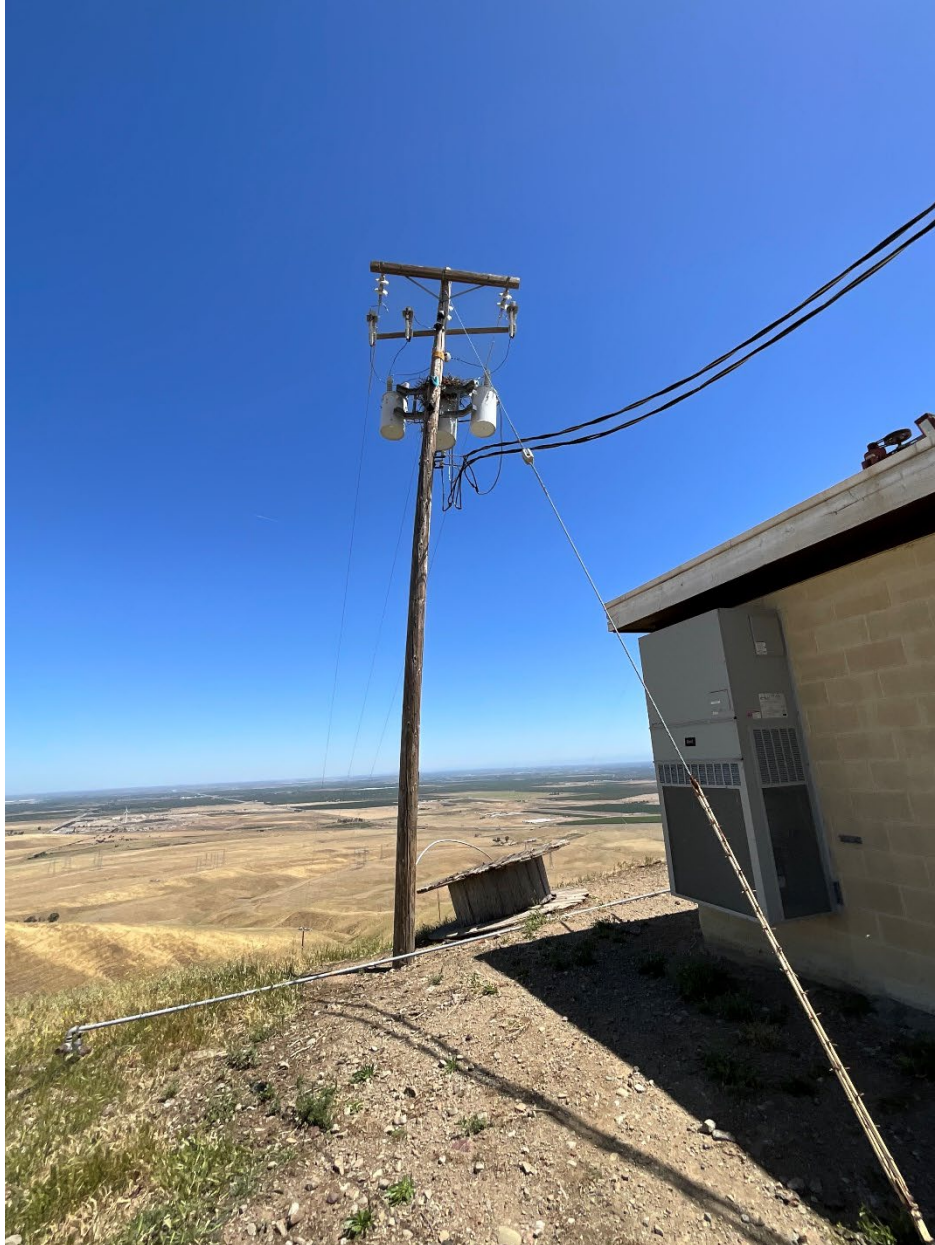
Figure 19: Wind Related Damage in San Joaquin County – Ground wire detached from pole and bird nest on pole
