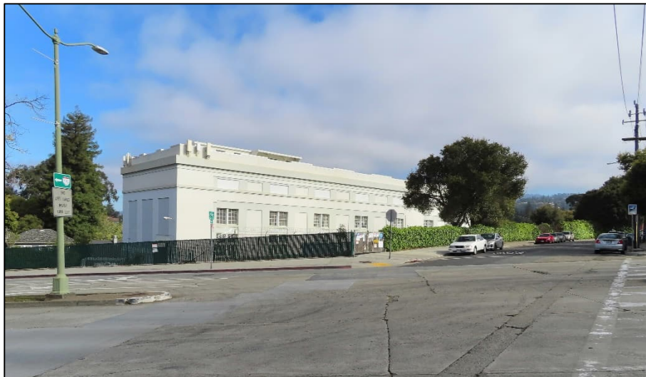
Photograph 2. Oakland X Substation, view north (Jacobs March 2024).
