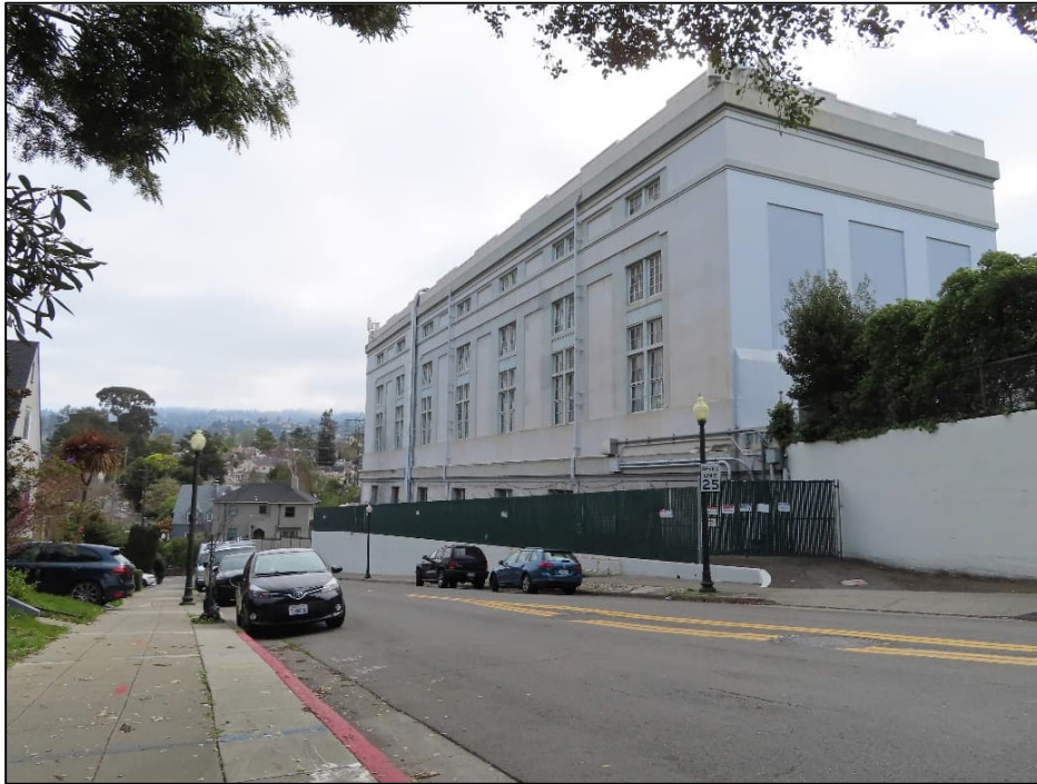
Photograph 1. Oakland X Substation, view east (Jacobs March 2024).
