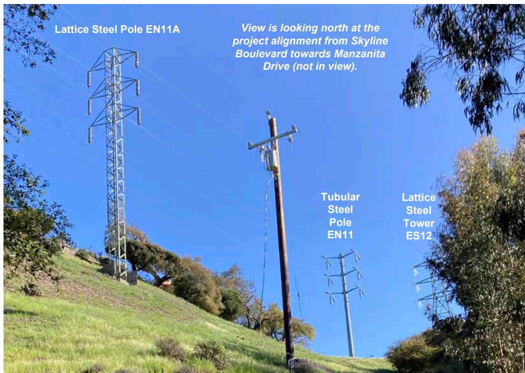
Figure 3.1-2a Existing Lattice Steel Towers, Tubular Steel Pole and Lattice Steel Pole Moraga-Oakland X 115 kV Rebuild Project Pacific Gas & Electric Company
