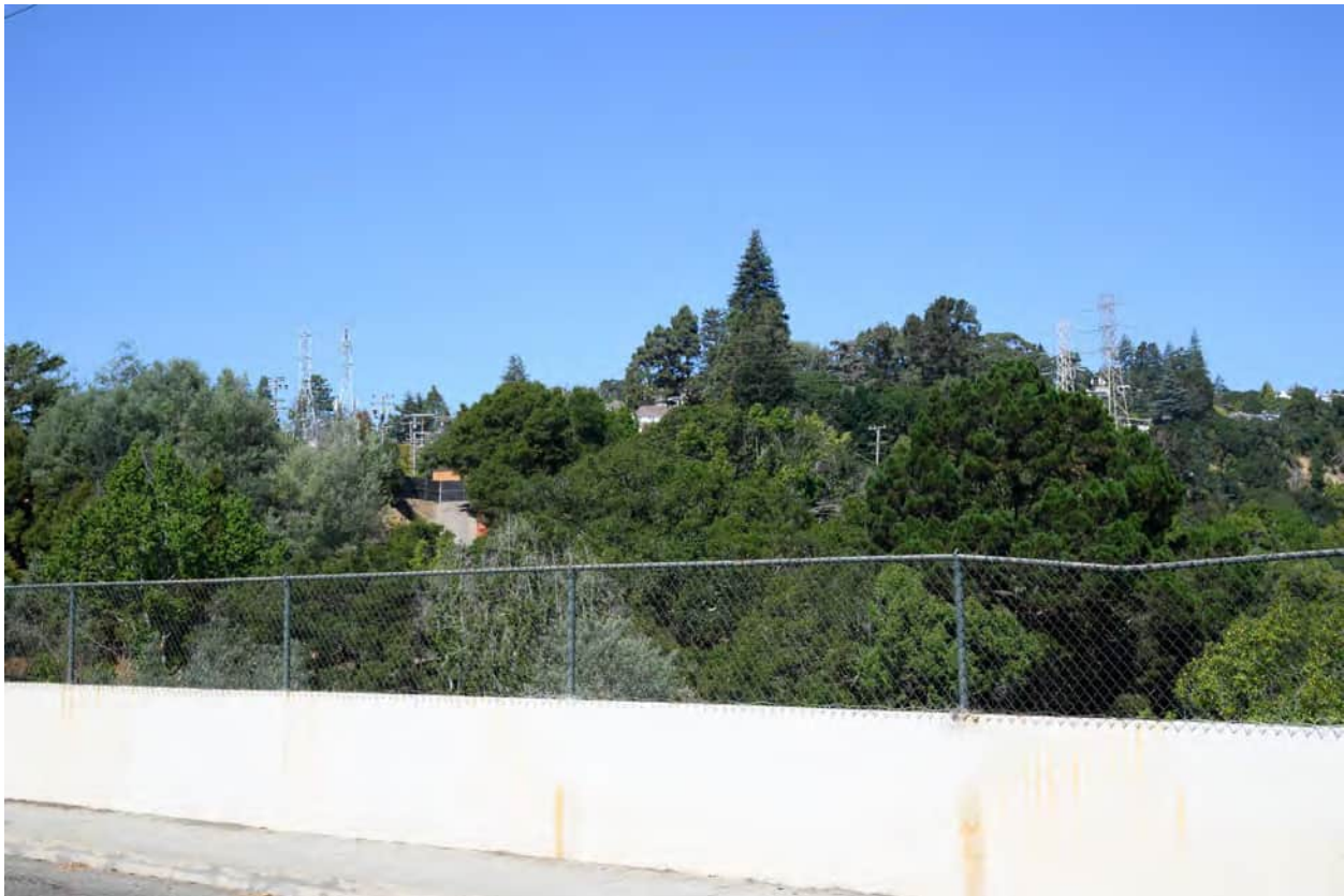
14. Leimert Bridge looking north Structures EN28, ES30 * KOP; see Figure 5.1-14 for visual simulation Refer to Figure 5.1-1a for photograph viewpoint locations
