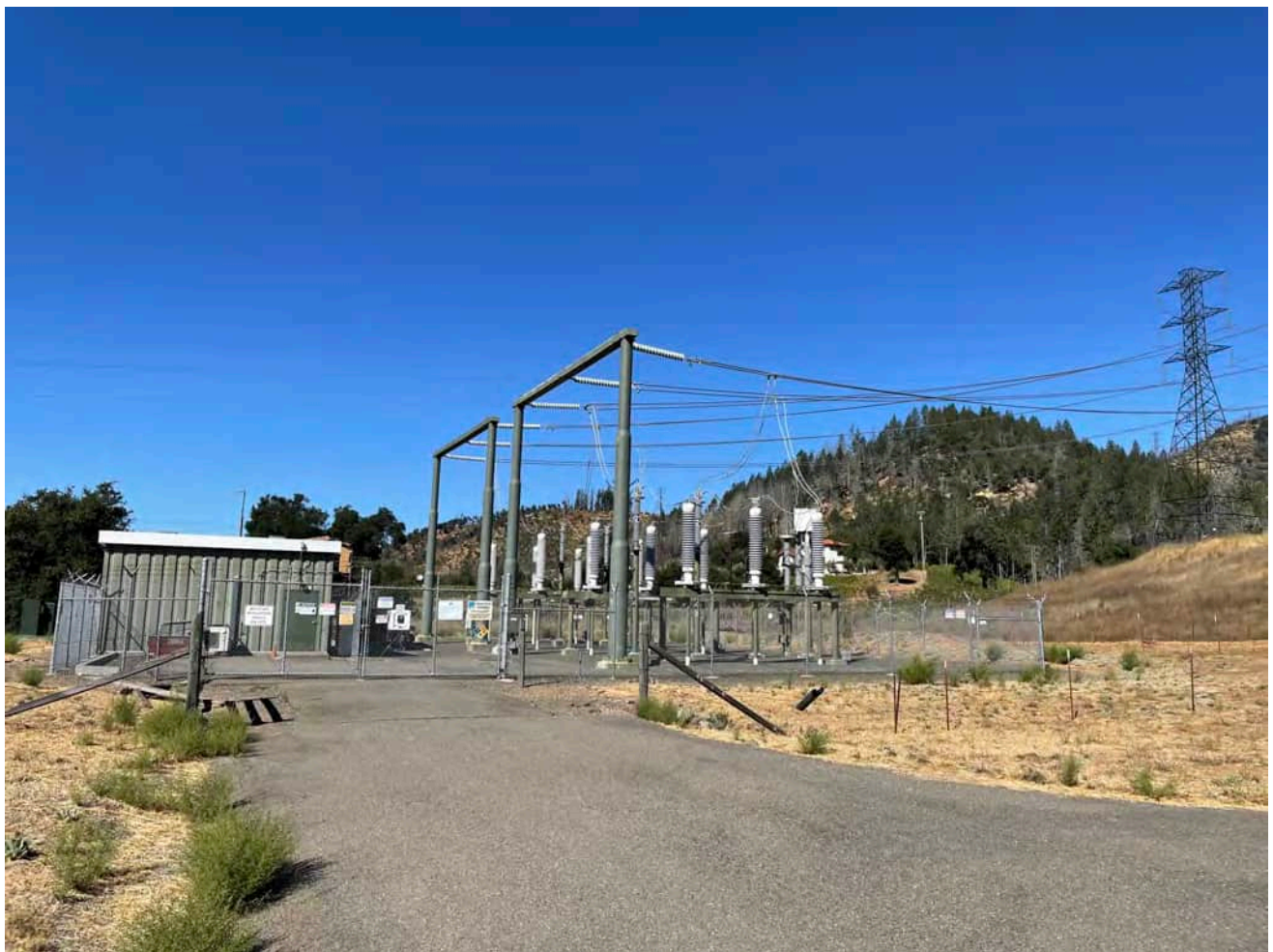
Figure 4.2-8 Example Transition Station with Two 230 kV Circuits in an Approximately 0.3-acre Yard Moraga-Oakland X 115 kV Rebuild Project Pacific Gas & Electric Company
