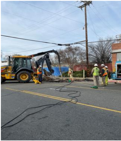
Figure 49 – PG&E's Maintenance & Construction Crew at Work
