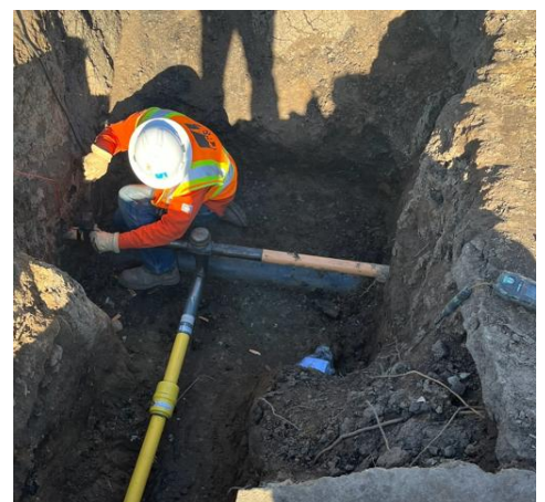
Figure 21 – Employee Working on Distribution Main and Service
