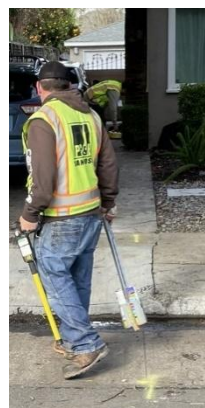
Figure 26 – PG&E Coworker Marking a Gas Main and Service
