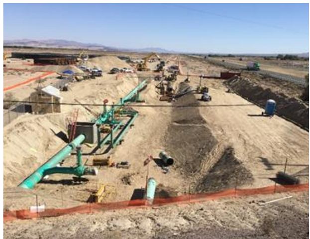
Figure 39 – Strength Test in Progress
