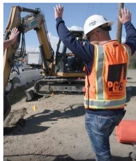
Figure 27 – Standby Crew at Work During Excavation
