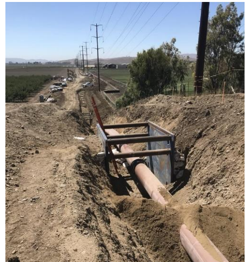
Figure 46 – L-301A Fault Crossing Pipe Replacement
