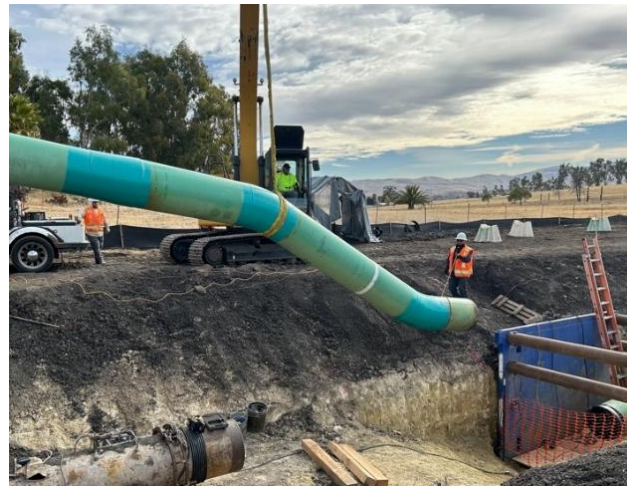
Figure 19 – Line 114 Retrofit Near Livermore
