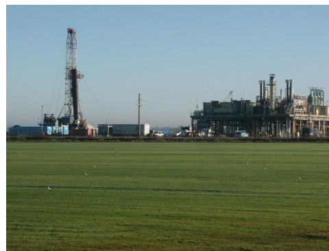
Figure 17 – Rig and Well Platform
