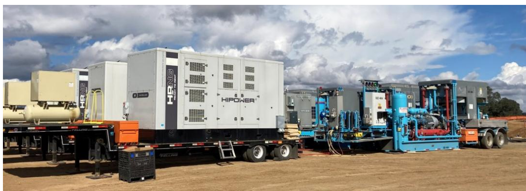
Figure 23 – Portable Cross Compression Degassing Isolated Segment of Pipeline into Adjacent Line
