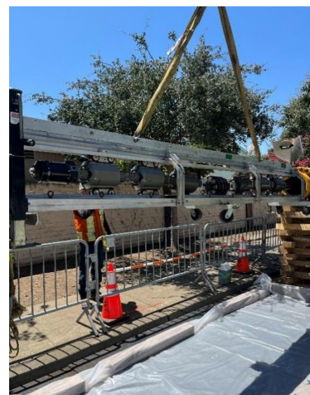
Figure 44 – 10" x 14" NT-ILI Tool Inspecting a 12" Pipeline
