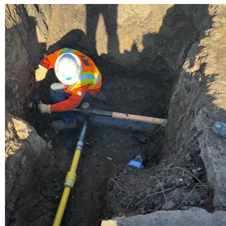
Figure 22 – Employee Working on Distribution Main and Service
