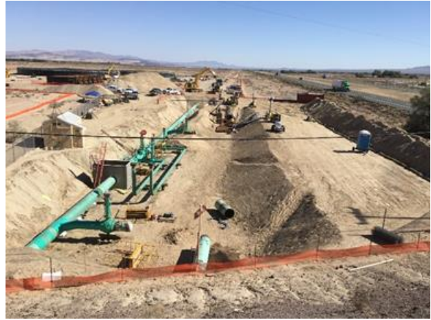
Figure 36 – Strength Test in Progress
