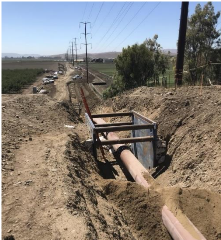
Figure 43 – L-301A Fault Crossing Pipe Replacement
