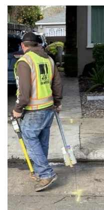
Figure 27 – PG&E Coworker Marking a Gas Main and Service
