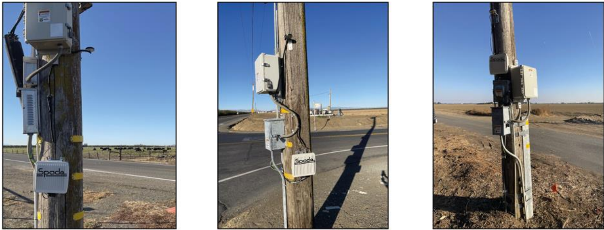
Figure 70 – SPADE demonstrating unit installed on PG&E Transmission Pipeline’s Cathodic Protection System network at Dixon in Q4 2024
