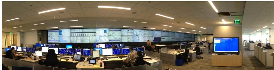
Figure 50 – PG&E's Gas Control Center Features a 90 Foot-Long Video Wall with Current Operational Information to Augment the Gas SCADA System
