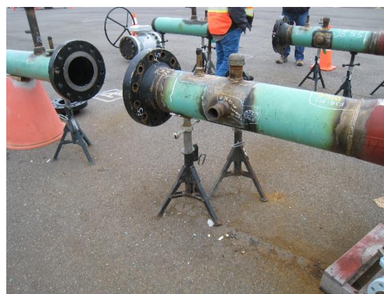
Figure 41 – Pigging training loop piping under construction
