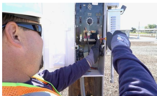
Figure 42 – PG&E Employee Installing a Cathodic Protection Rectifier
