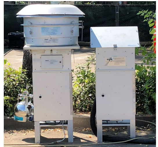
Air monitoring equipment will be used to confirm the work is done in a health protective manner.
