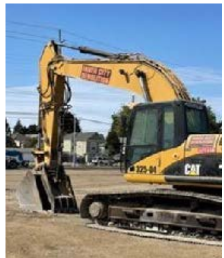
Excavators and other heavy equipment will be used to remove soil.
