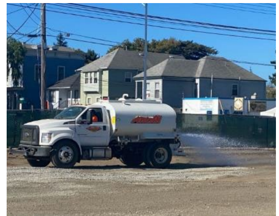
Soil will be kept damp to help control dust and odors.
