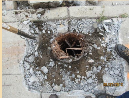
After extraction showing below ground deterioration
