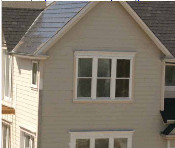
Figure 4-16. OCR Solar Solutions roofing material, http://www.oldcountryroofing.com
