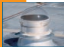
Tubular skylight with clear plastic dome.
