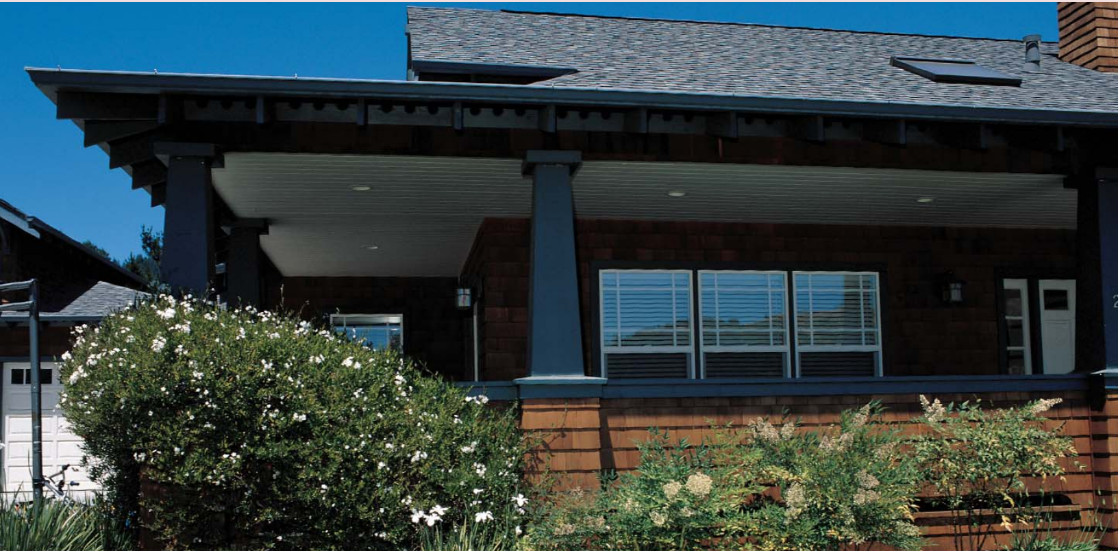
Properly-designed architectural features, such as overhangs and trellises, help keep out the hot summer sun yet allow the sun to warm your home in winter.
