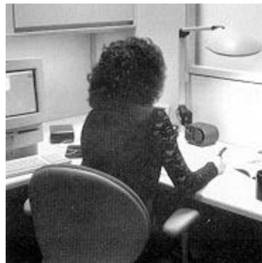
Individual workstation with direct lighting and task lighting.
