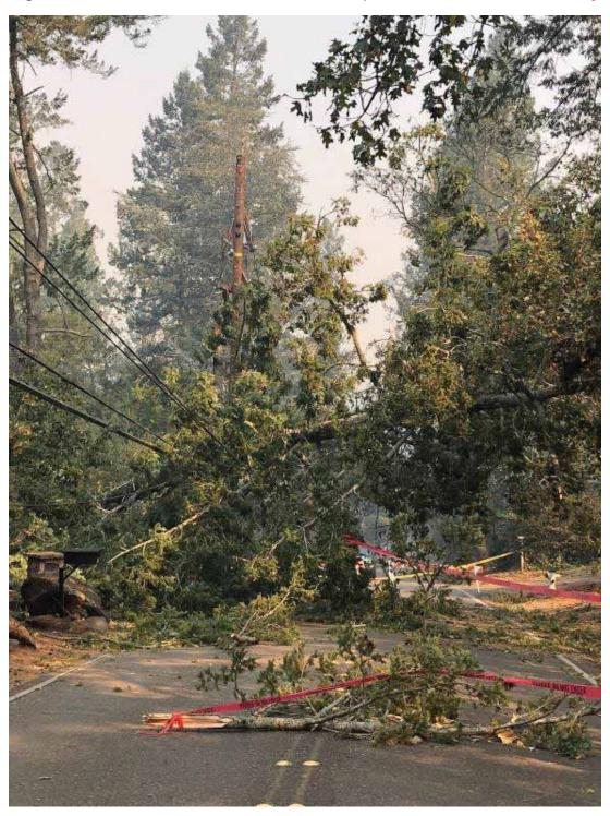
Figure 4: Tree fell on to conductors in Oakland, Alameda County
