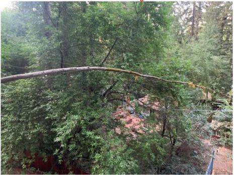
Figure 16 – In Boulder Creek, Santa Cruz County Branch in Contact Cross Phase Conductors
