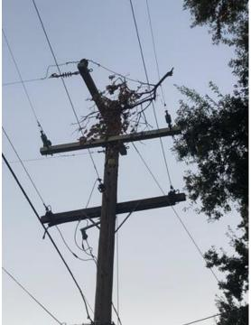
Figure 4 – In Calistoga, Napa County Branch Flew Into Primary Conductors
