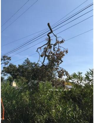
Figure 5 – In Cottonwood, Shasta County Branch Flew Into Primary Conductors
