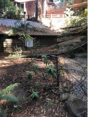
Figure 2 – In Artois, Glenn County Branch Fell Onto Secondary Conductors Bringing Down the Lines
