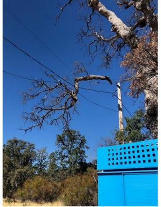
Figure 8 – Near Redding, Shasta County Tree Failed Onto Primary Conductors and Took Down Pole
