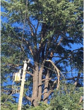
Figure 7 – In Stonyford, Colusa County Branch Flew Into Secondary Conductors
