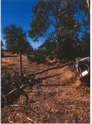
Figure 3 – In Los Molinos, Tehama County Branch Flew Into Primary Conductors
