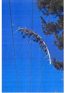
Figure 6 – In Red Bluff, Tehama County Branch Failed Into Primary Conductors
